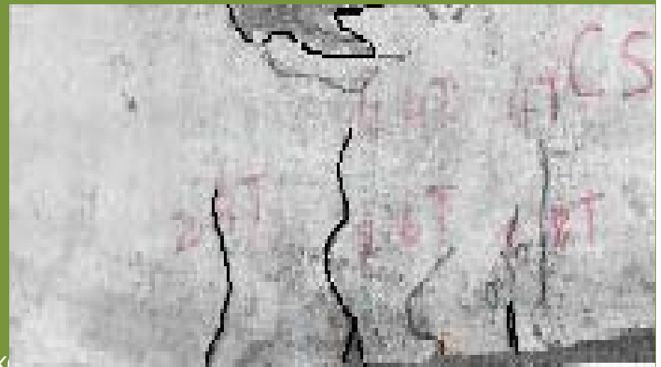
Fig d. Transverse crack in beam
