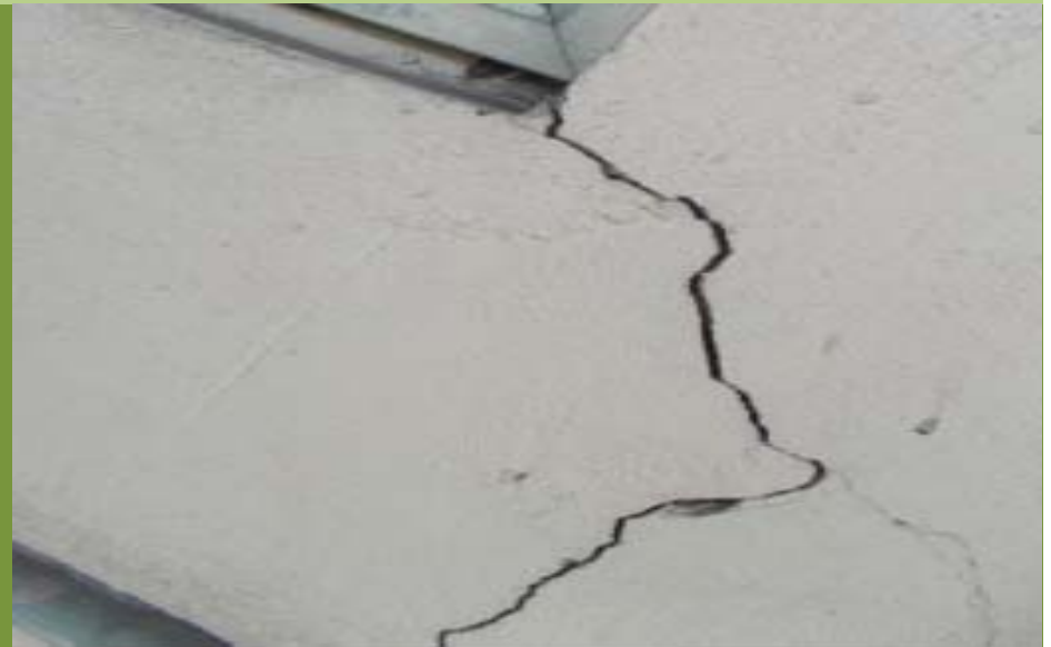
Fig b. Diagonal crack in Wall from opening
