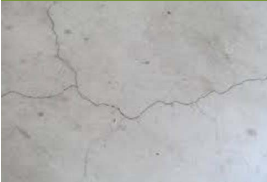
Fig c. Random crack in Floor slab
