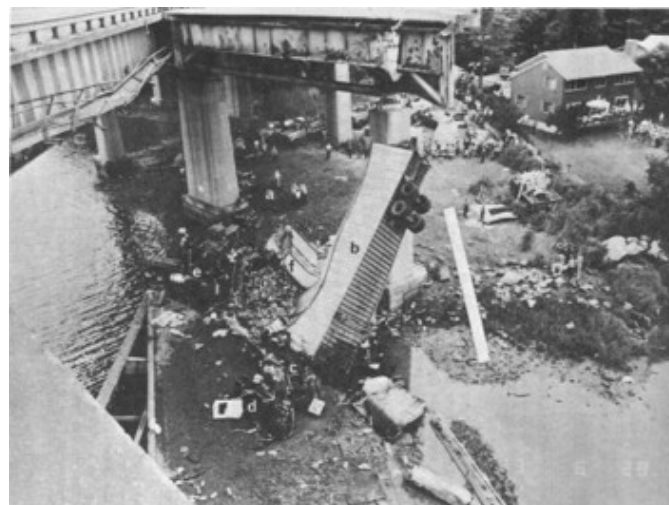
Figure 31.18. Mianus River Bridge collapse (NTSB 1984).
