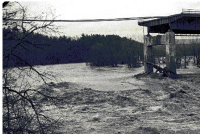
Figure 31.17. Schoharie Creek Bridge pier collapse (USGS, 1997).
