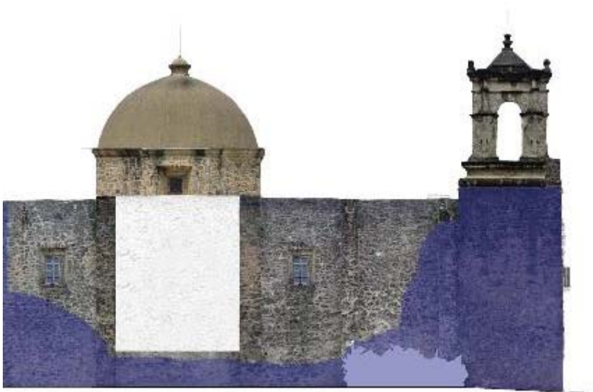
Northern photo elevation: In blue - original walls
