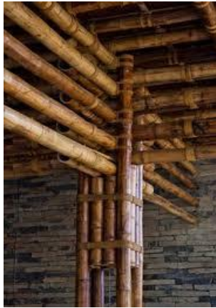
Fig. 7. Beam Column Joint
