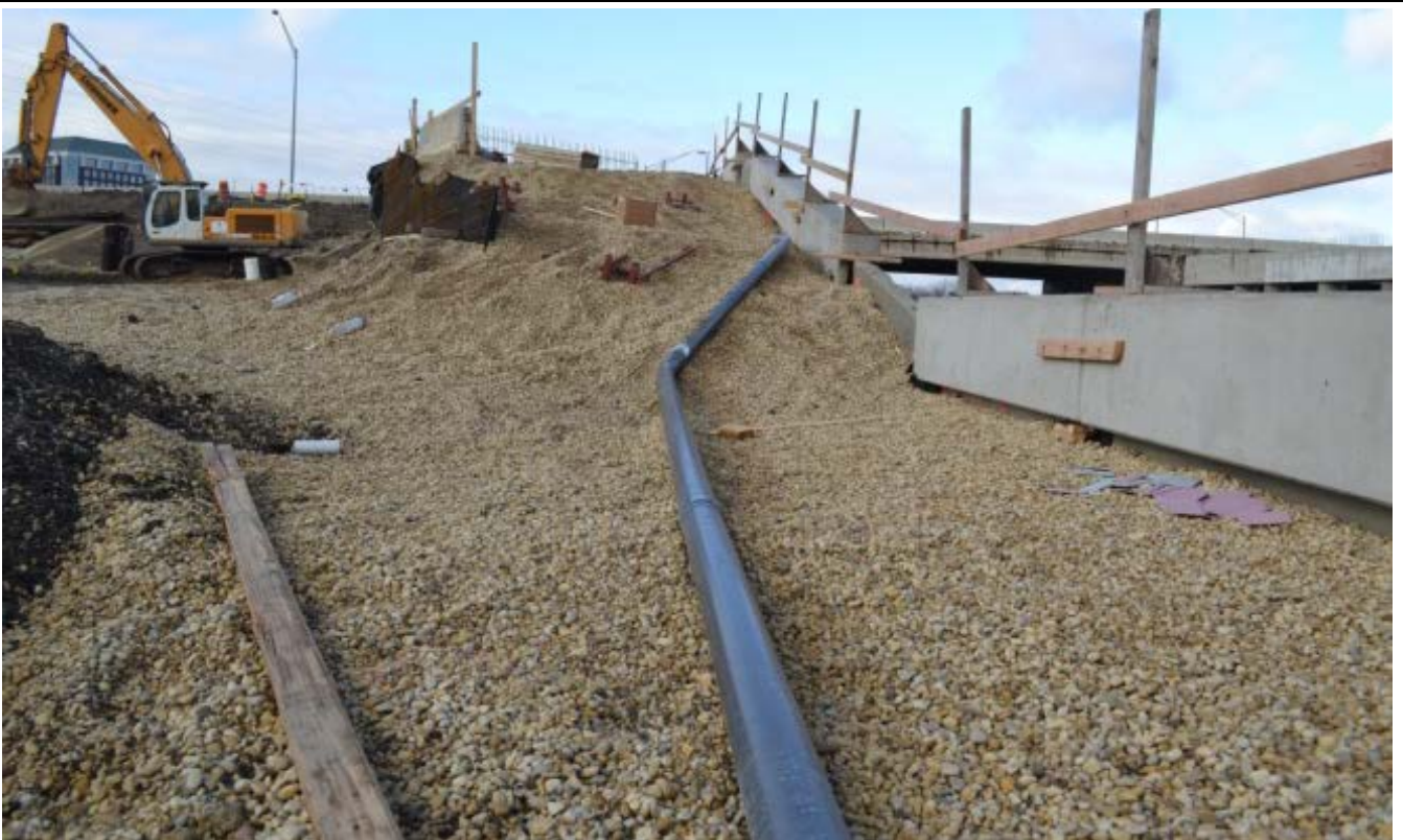
Drainage pipe to relieve pressure from water build-up.
