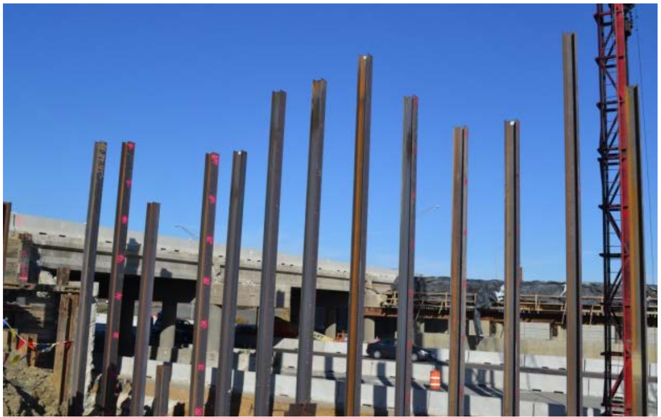
These piles are all the same length and driven to the correct bearing depth.
