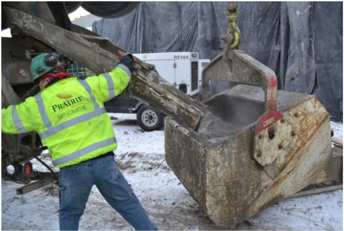
Filling a 2 yard concrete bucket. The concrete from this truck was tested by both the QA and QC Inspectors.
