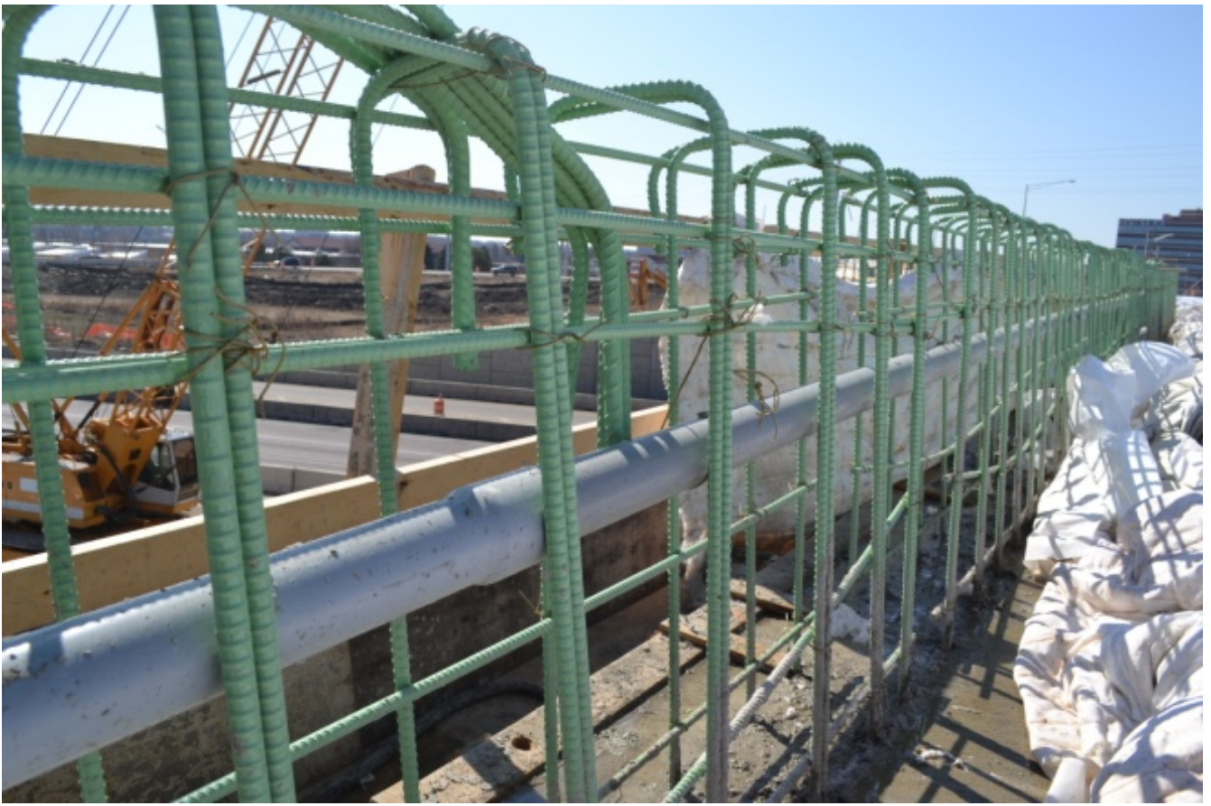
Re-bar and electrical conduits were installed before concrete was poured.
