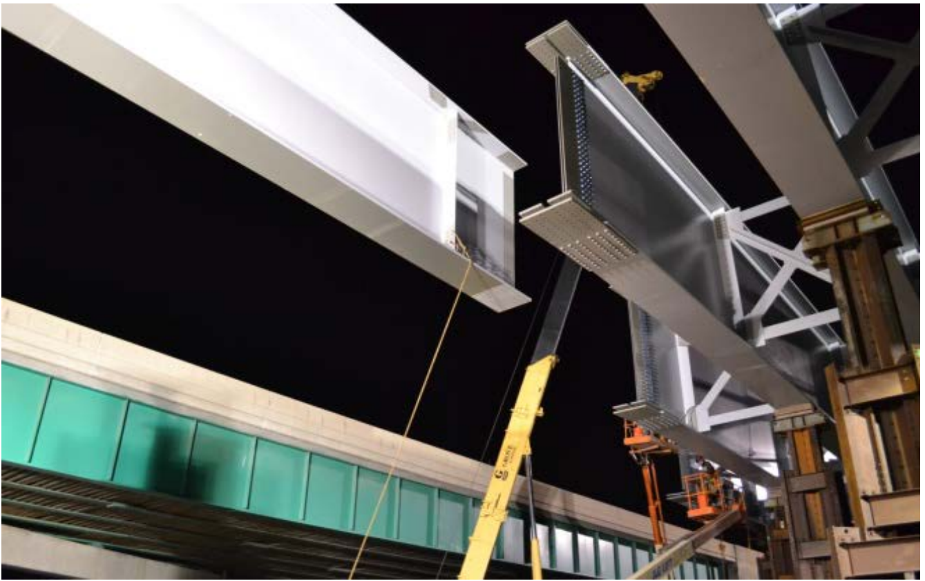
Raising a beam and getting close to the splice.
