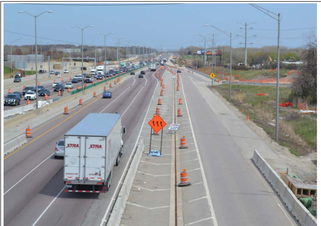
Barrels, signs, and temporary barrier walls placed to properly weave traffic around center pier construction.
