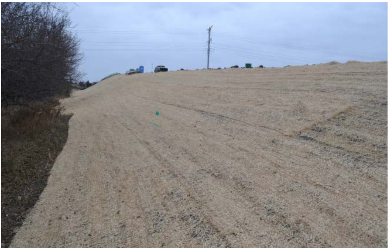
Seed and erosion control blanket on the finished slope. The CM Team verified the proper slope and measured and paid for this work.
