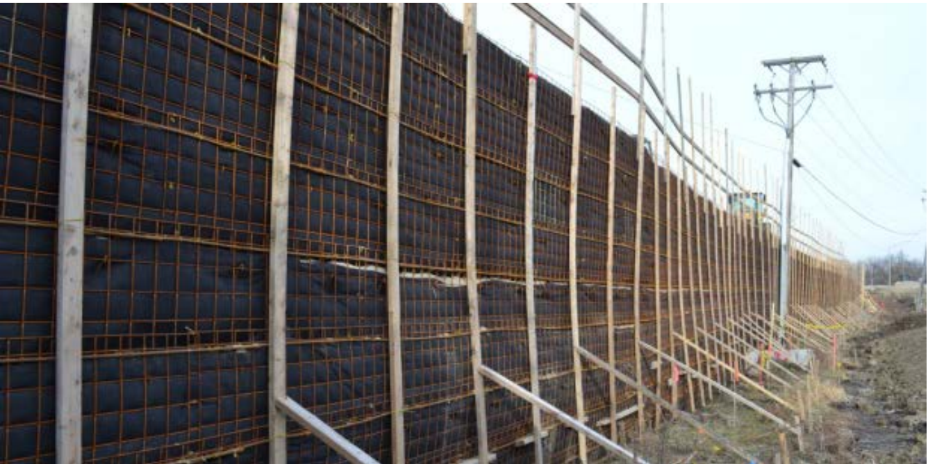
Temporary MSE Wall completed in 18 inch baskets.
