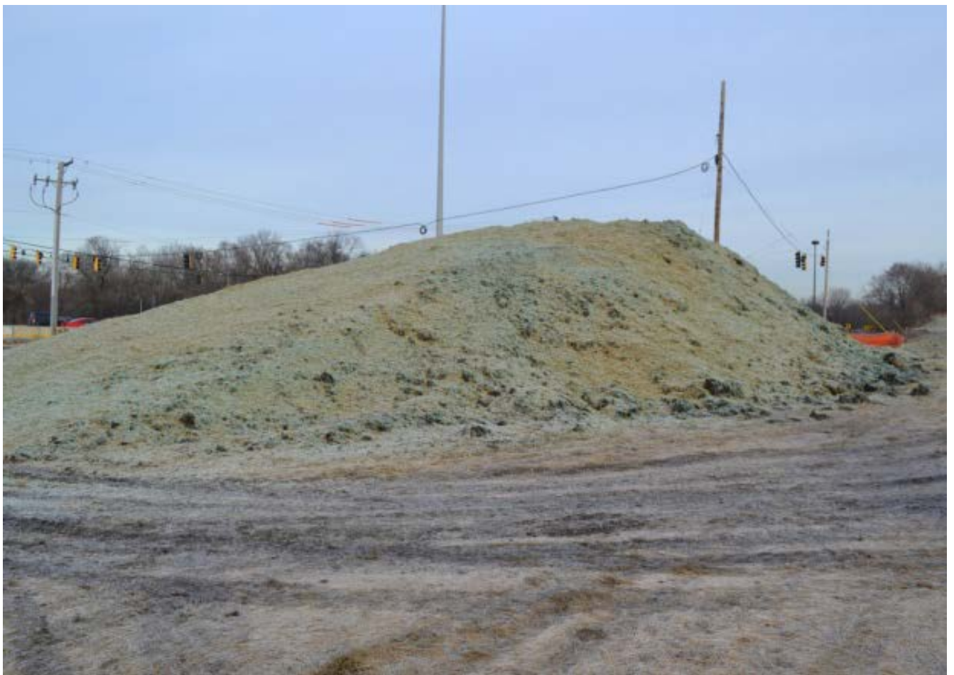
Topsoil stockpile with temporary seeding and erosion control blanket.
