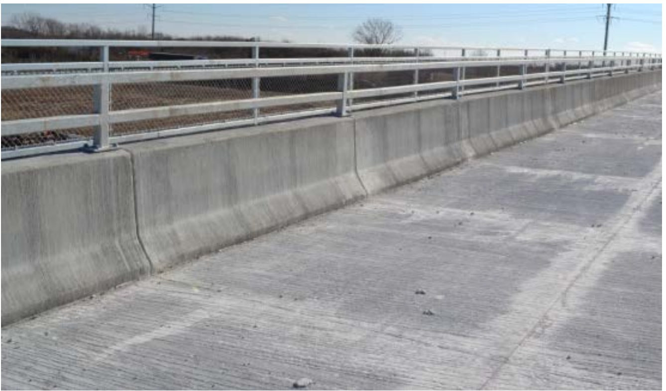
The finished parapet wall with a pedestrian railing.
