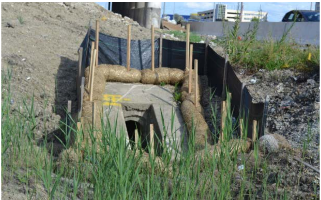
Silt fence and ditch checks protected an existing drainage structure.
