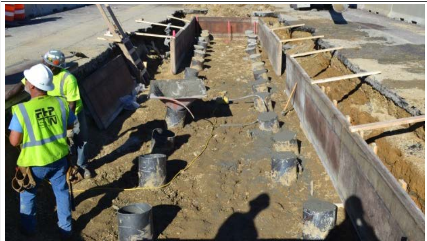
Shell cast in place pipe piles, cut off, and being filled with concrete.
