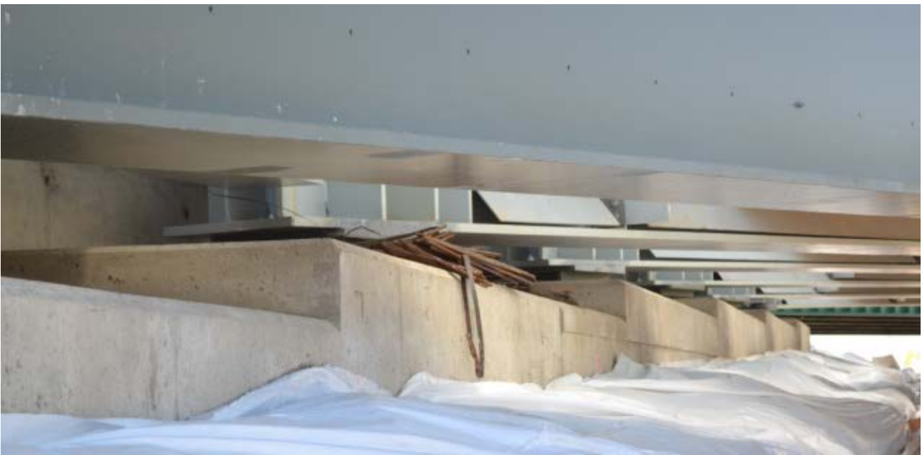
Detail of stepped abutment.
