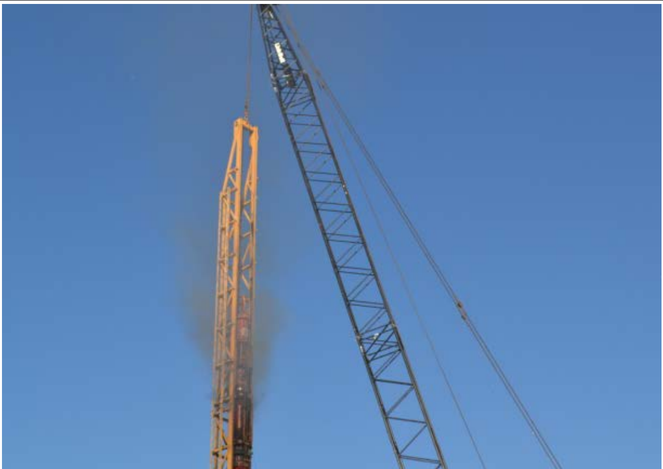
Diesel hammer firing to raise and drop the hammer to drive the pile. The yellow structure is a heavy duty cage to enclose the pile and keep it straight.
