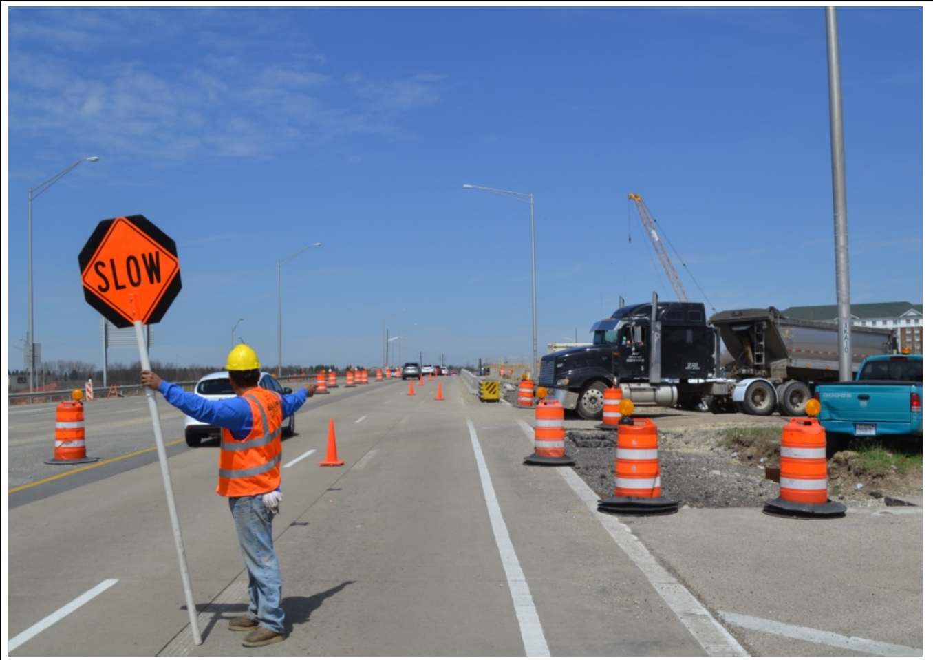
Flagger properly coordinating public traffic with construction traffic exiting onto a public road.
