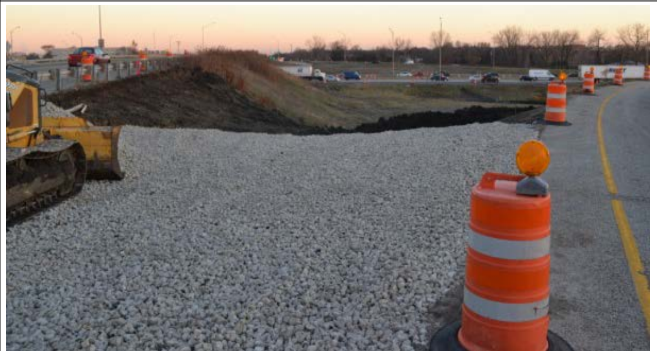
Stabilized construction entrance properly protected with traffic control barrels.
