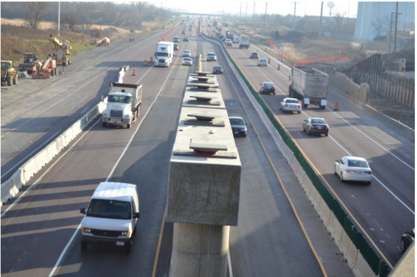
Center pier with fixed bearings. The beams will sit on these bearings. Surveyors have already verified the horizontal and vertical location of these bearings.
