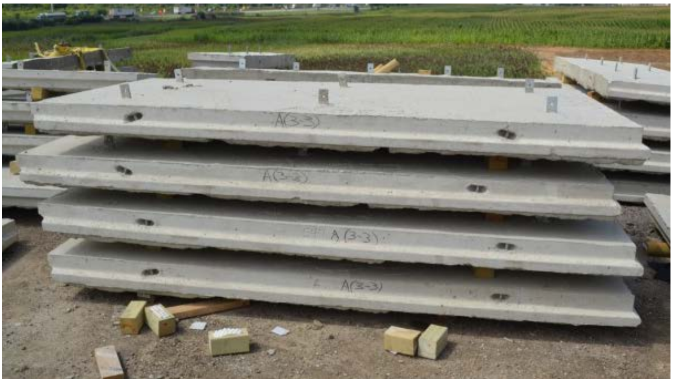
MSE Wall panels ready for installation.
