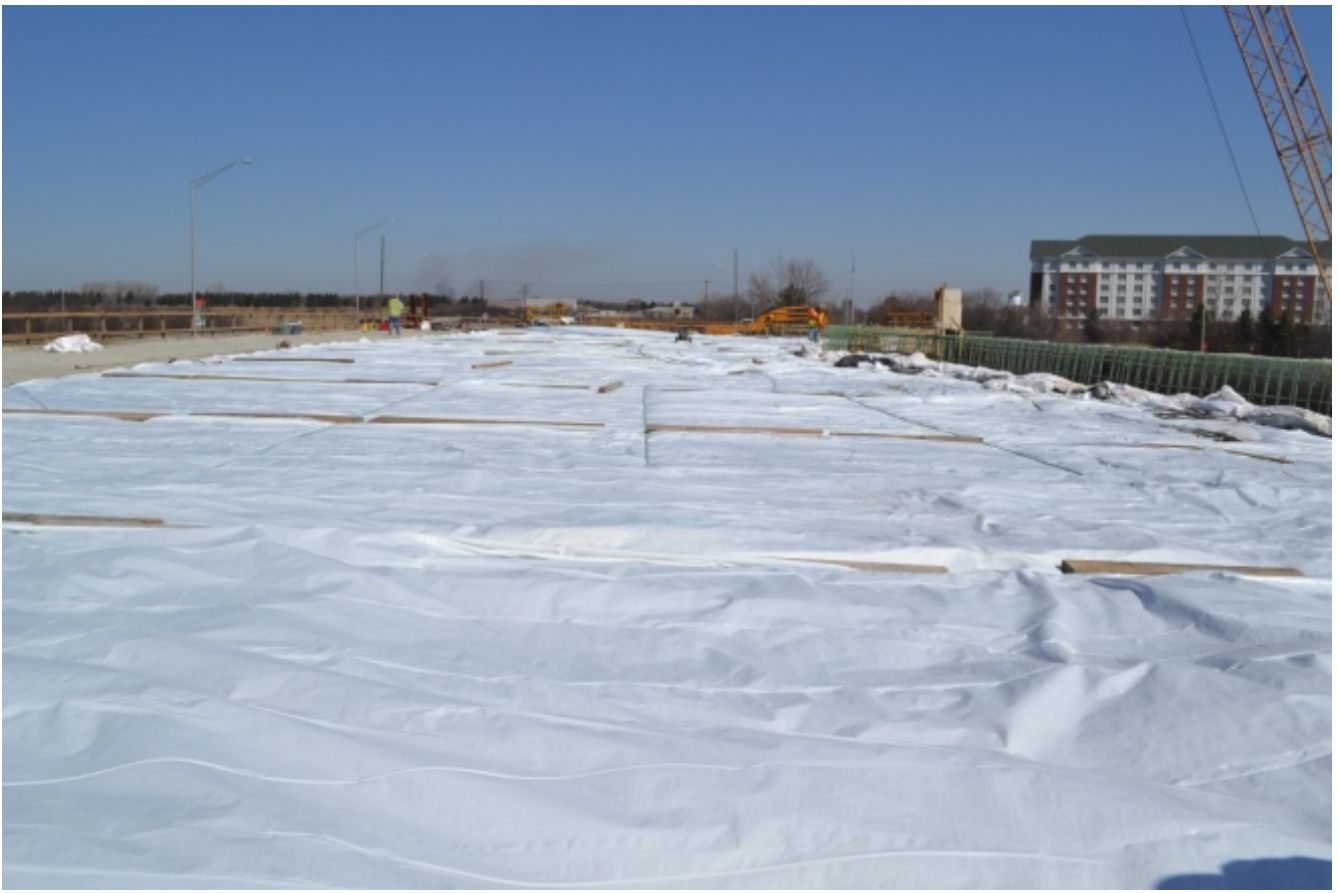
The fresh concrete was covered to properly cure for a minimum of 7 days.
