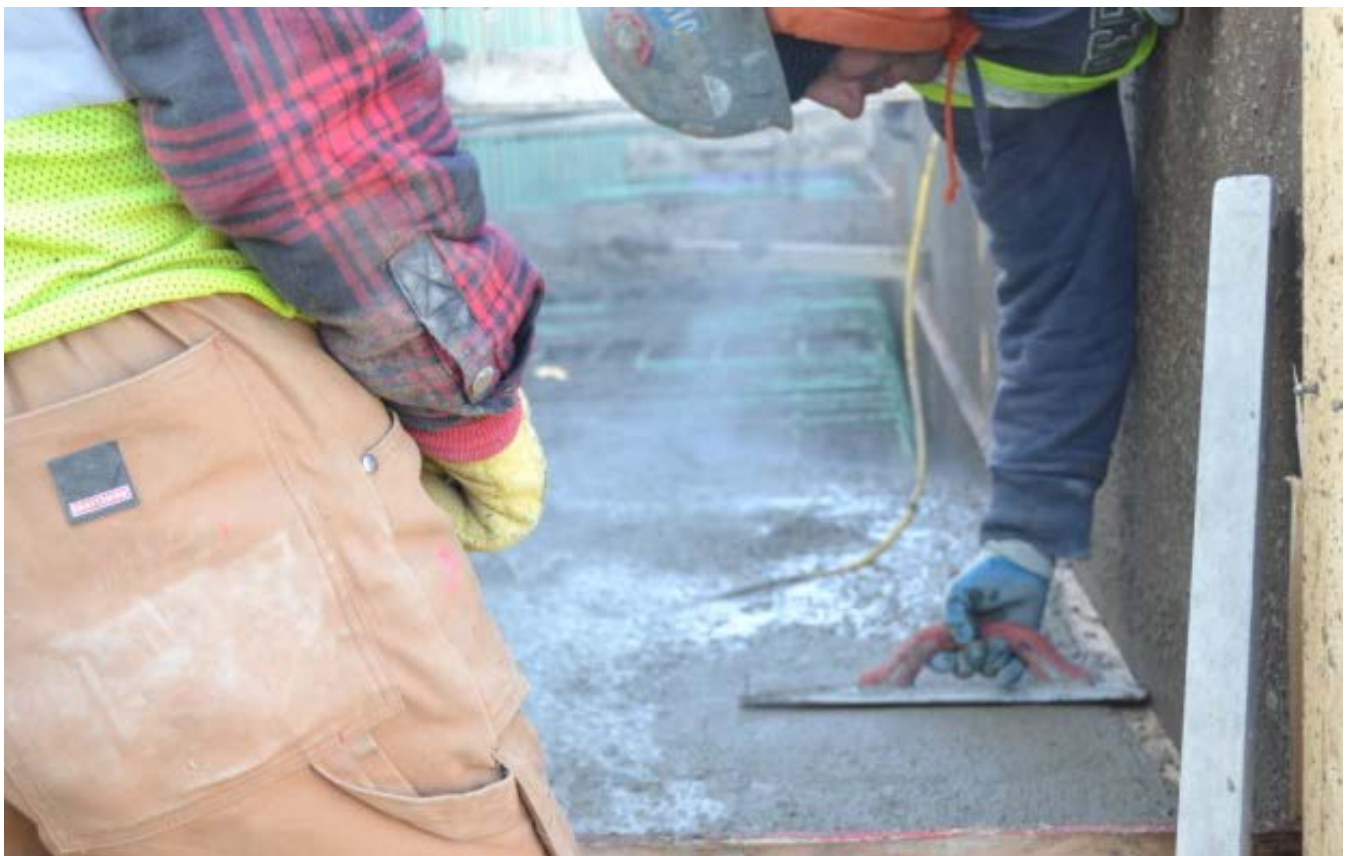
Finishing concrete for the abutment.
