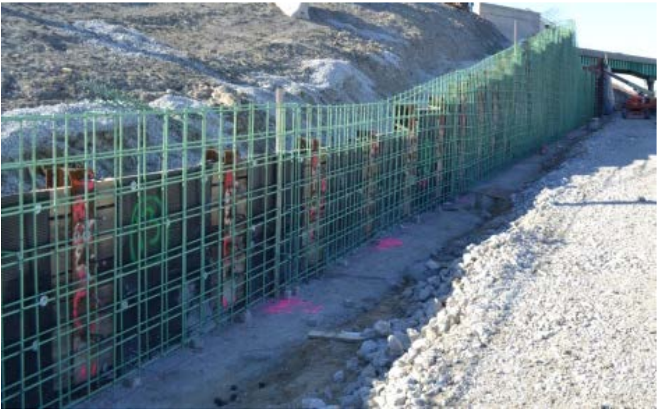
Re-bars in place ready for forms. The CM Team verified and measured the re-bars for payment.
