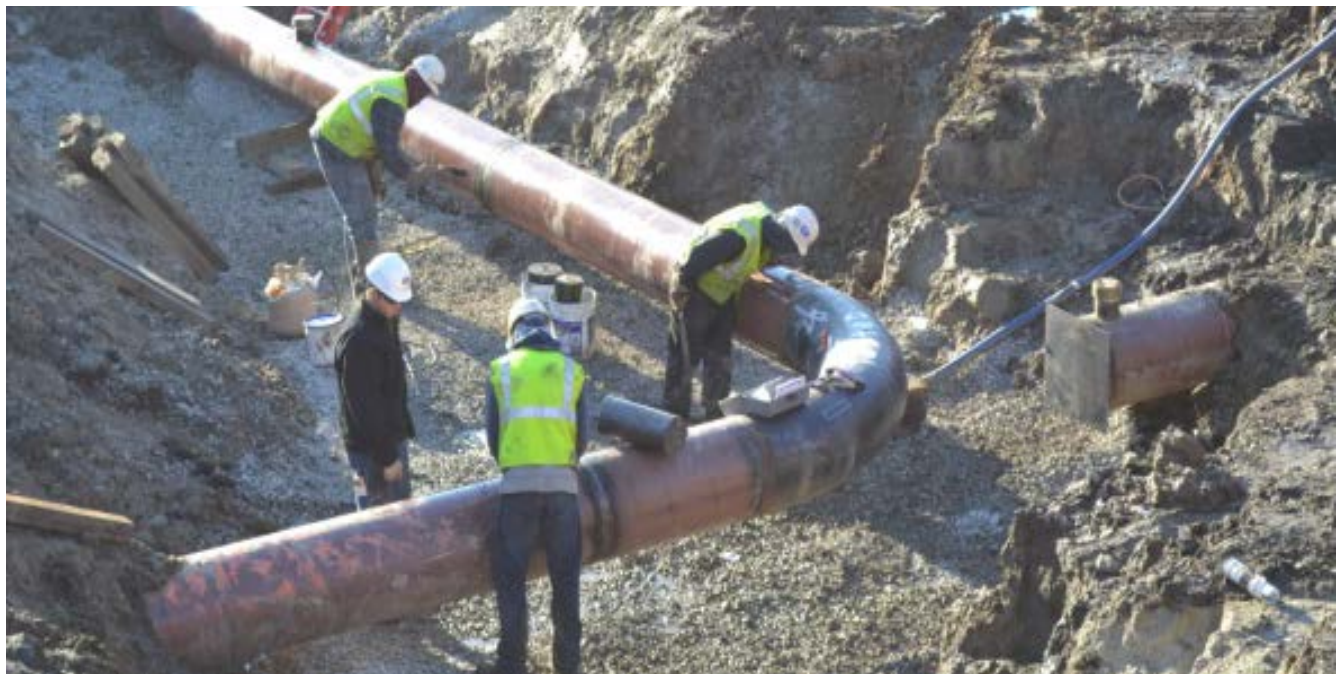
Gas pipeline being relocated. Engineers will test the welds prior to activating the line. Surveyors will mark the new route and verify that it was properly relocated. The CM Team will mark the new location on the as built plans.
