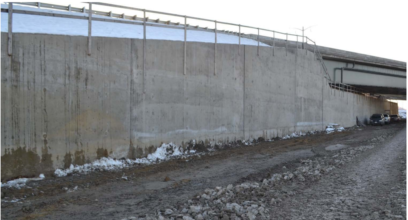
Completed Structural Concrete Wall with Footing.
