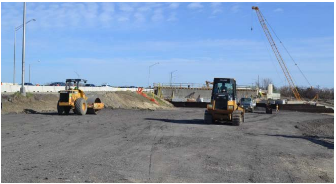
Beginning to place, grade, and compact FE. Both QA and QC Inspectors check the density of the compacted, in place, material.
