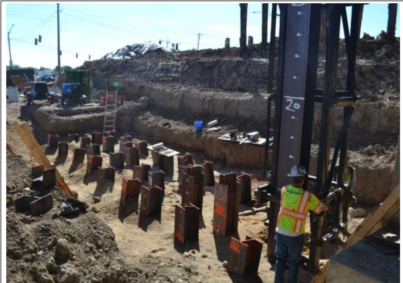
H-piles at center pier cut off at the correct final elevation.
