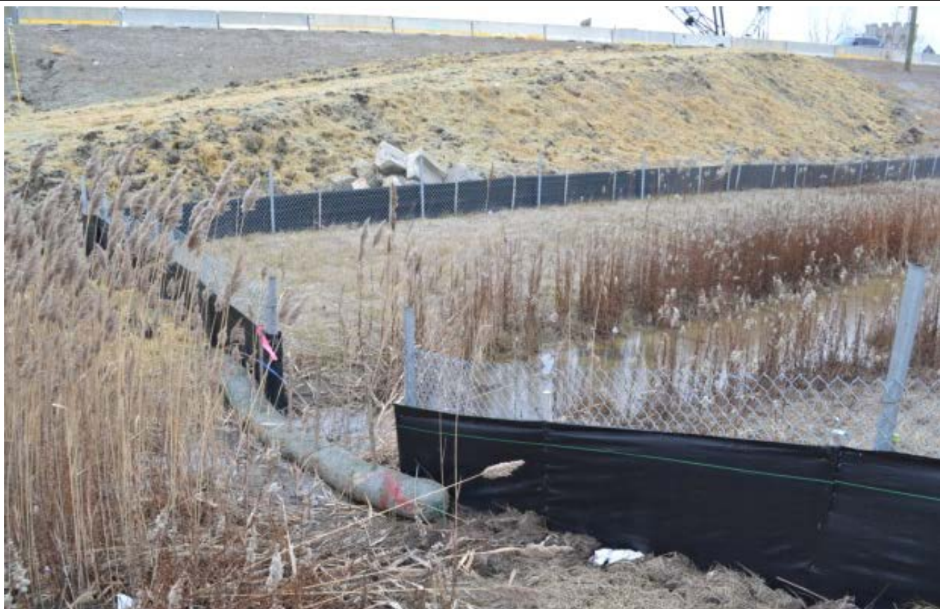
Wire reinforced fence provided extra stability to the silt fence.
