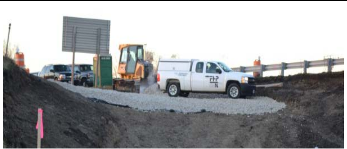
Topsoil was stripped, the subgrade was properly graded and compacted, and aggregate was placed.
