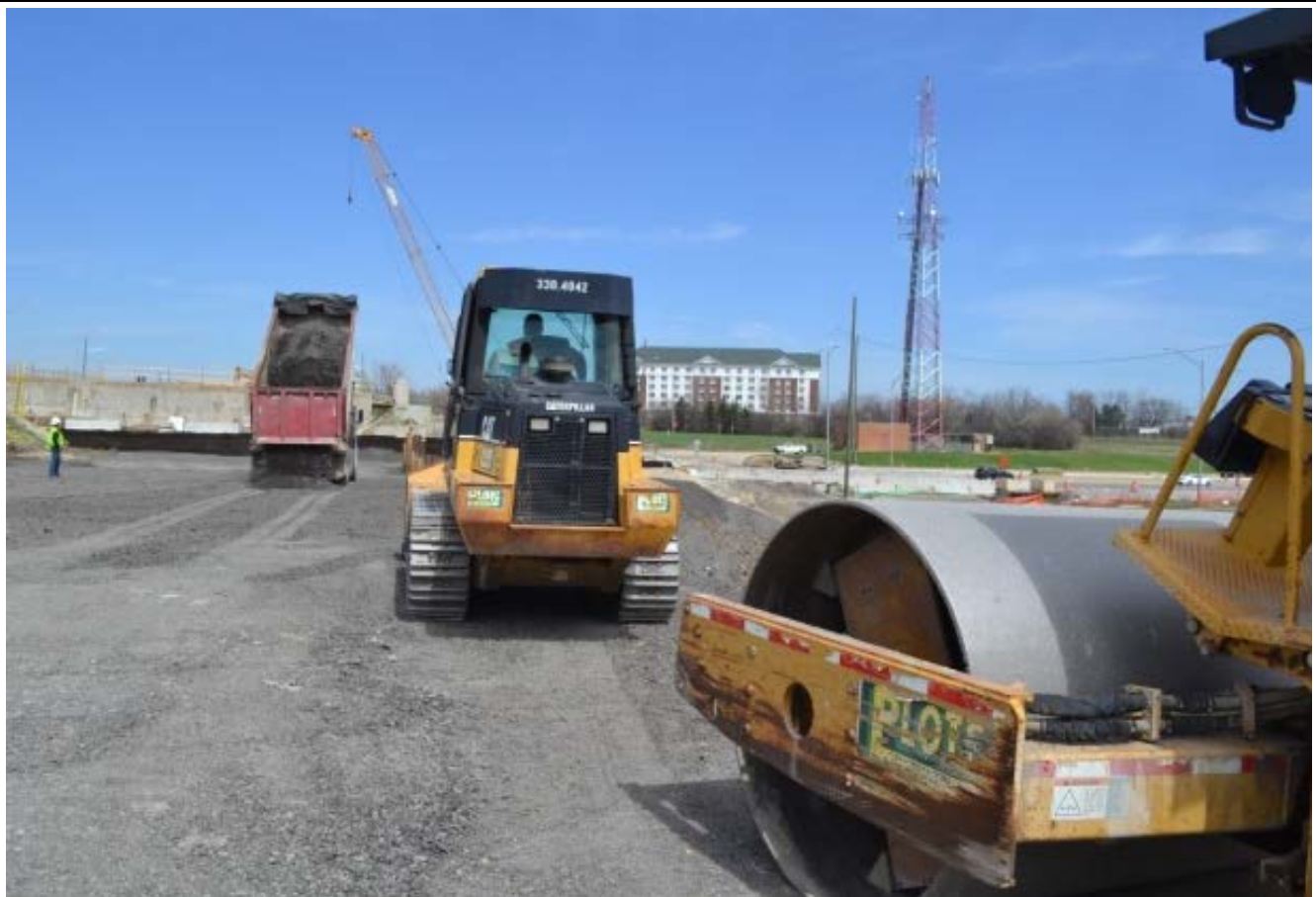
An 18 wheel semi-trailer, rear dump, can haul about 14 cu. yd. of material. Some locations required a very small amount but some required over 15,000 cubic yards of FE. A dozer spread the FE and a combination wheel/drum roller compacted it.
