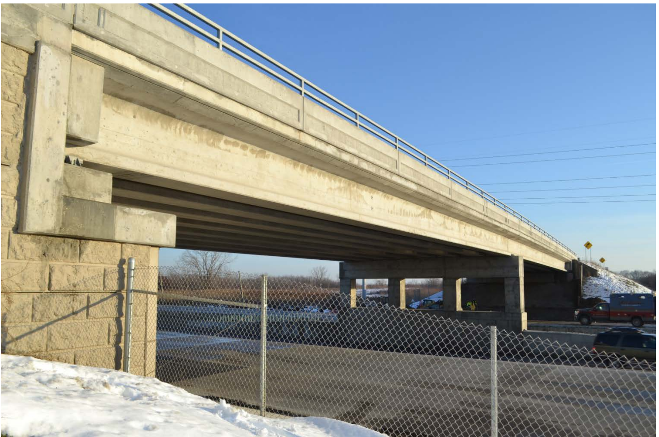
A typical, two-span bridge with abutments, a center pier, permanent retaining walls at the ends and along the sides, concrete beams to span the pavement, and a concrete deck with wearing surface for the vehicles to ride on.
