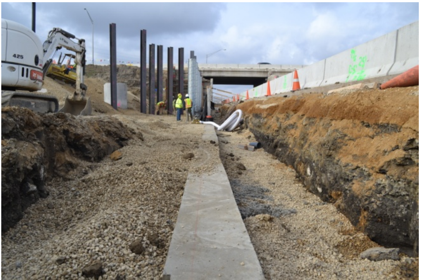
Footing for MSE Wall. A surveyor staked the horizontal and vertical position for the contractor to construct.
