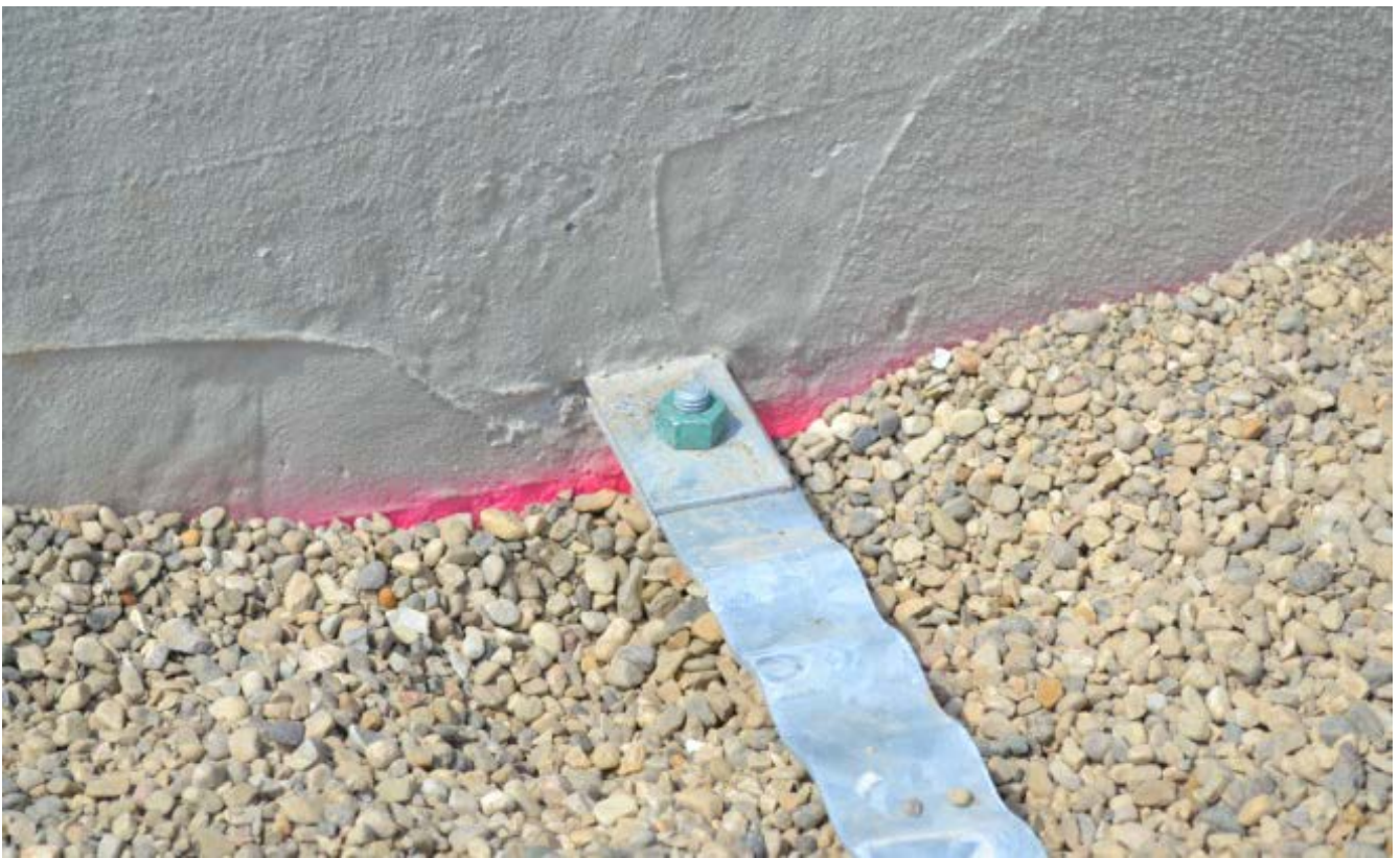
Tieback strap connection detail. This select backfill is called "Pea Gravel".
