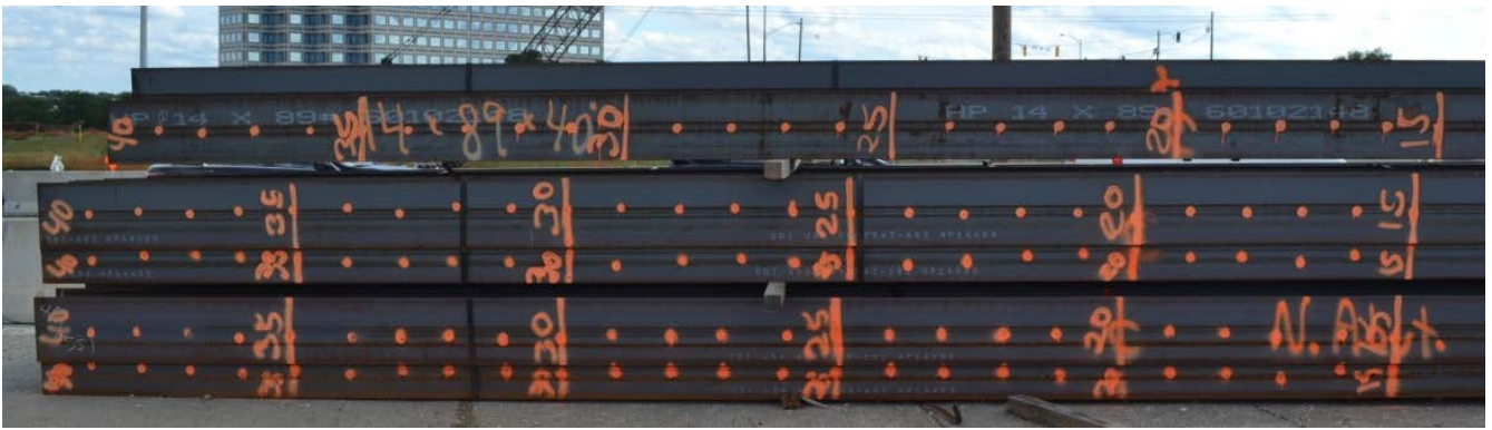
Stockpiled H-piles marked at 1 foot intervals by the contractor's field engineer and ready for installation.
