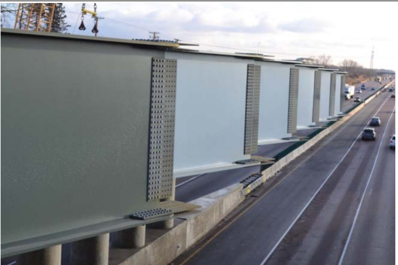
End of beams awaiting extension and proper connection.
