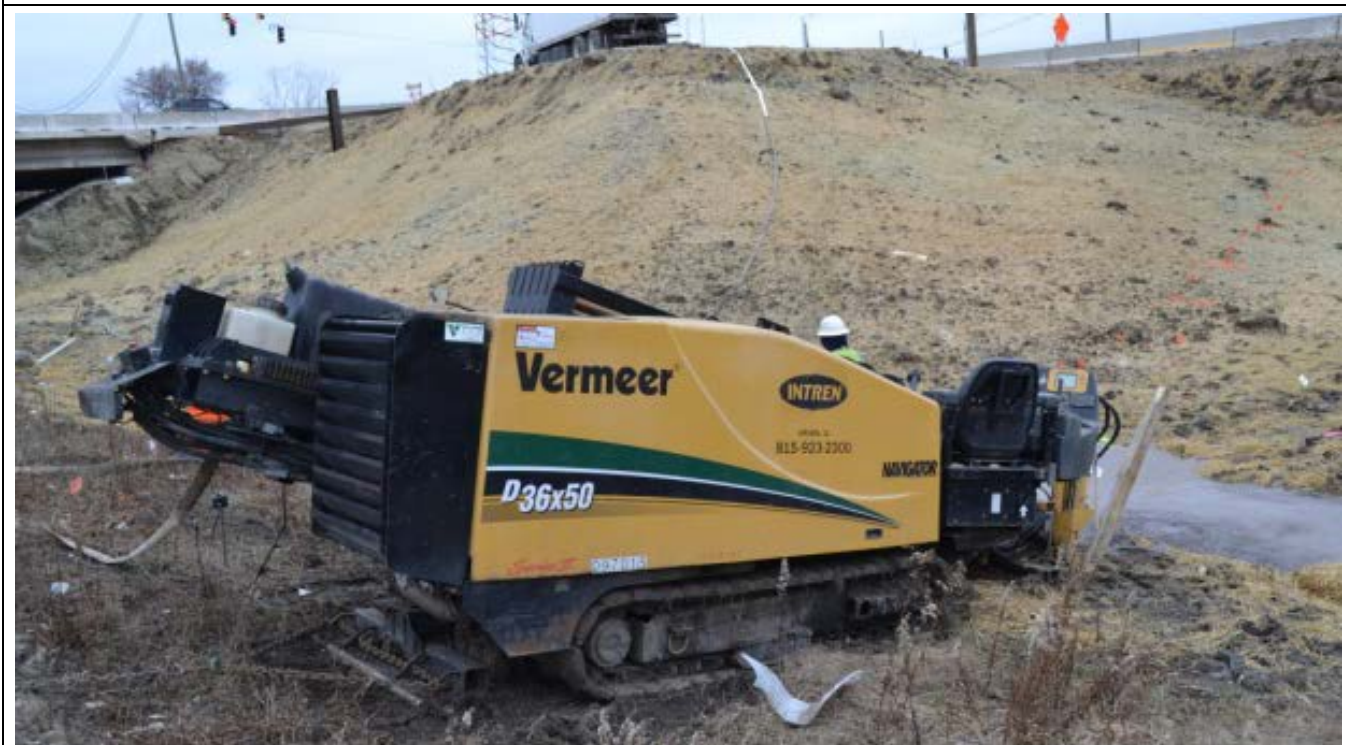
Direct bore machine relocating underground electric cables.
