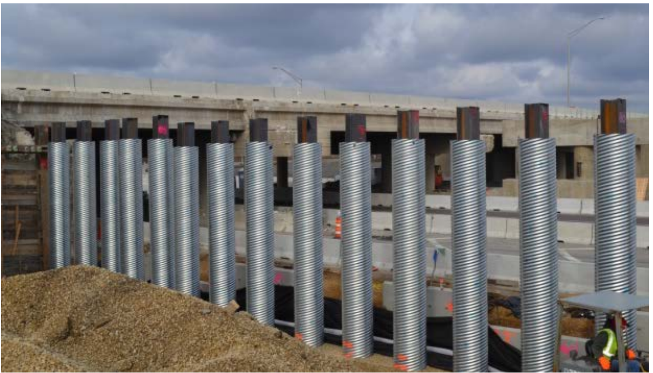
H-piles cut off at finish elevation in an abutment. Pile casings are visible before select backfill was placed around them.
