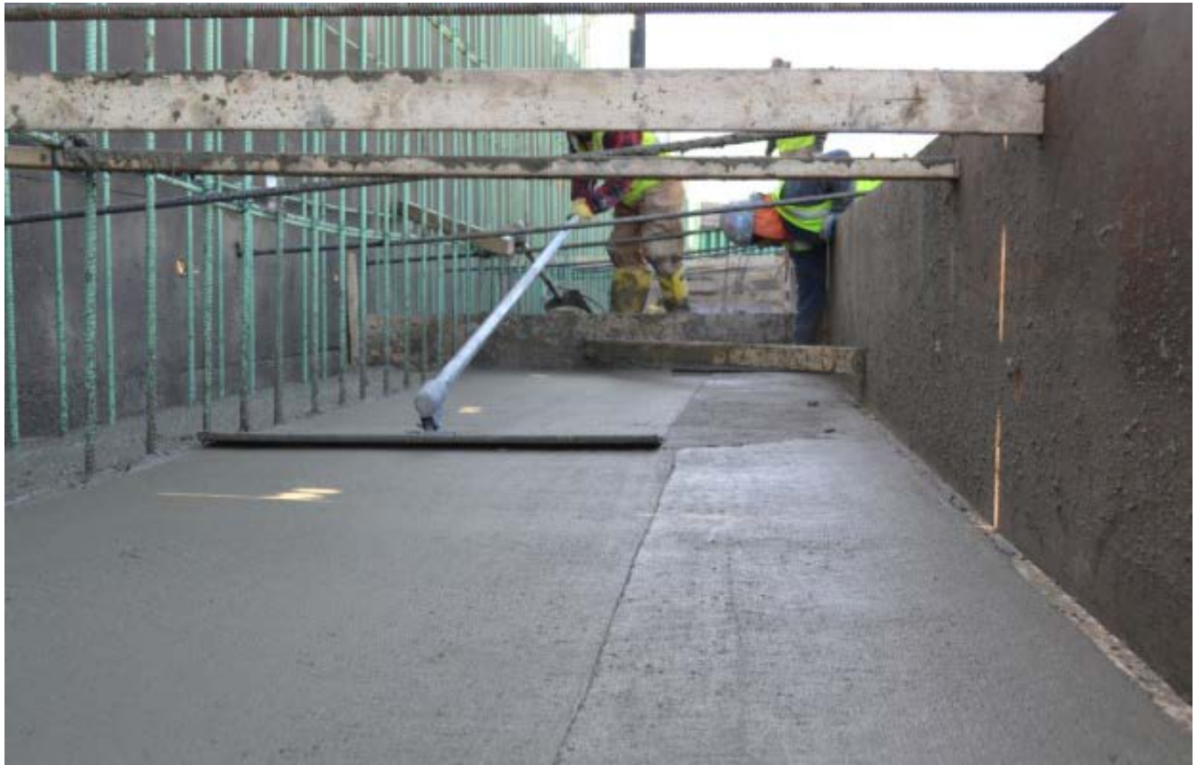
Finishing concrete for the abutment.
