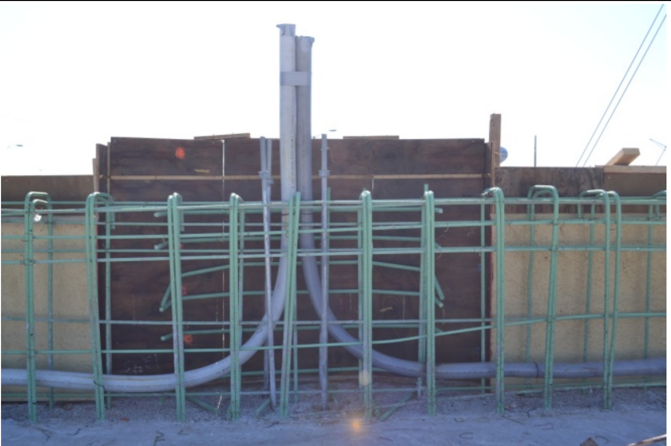
Conduit for lighting and message boards was designed and inserted into the barrier wall.
