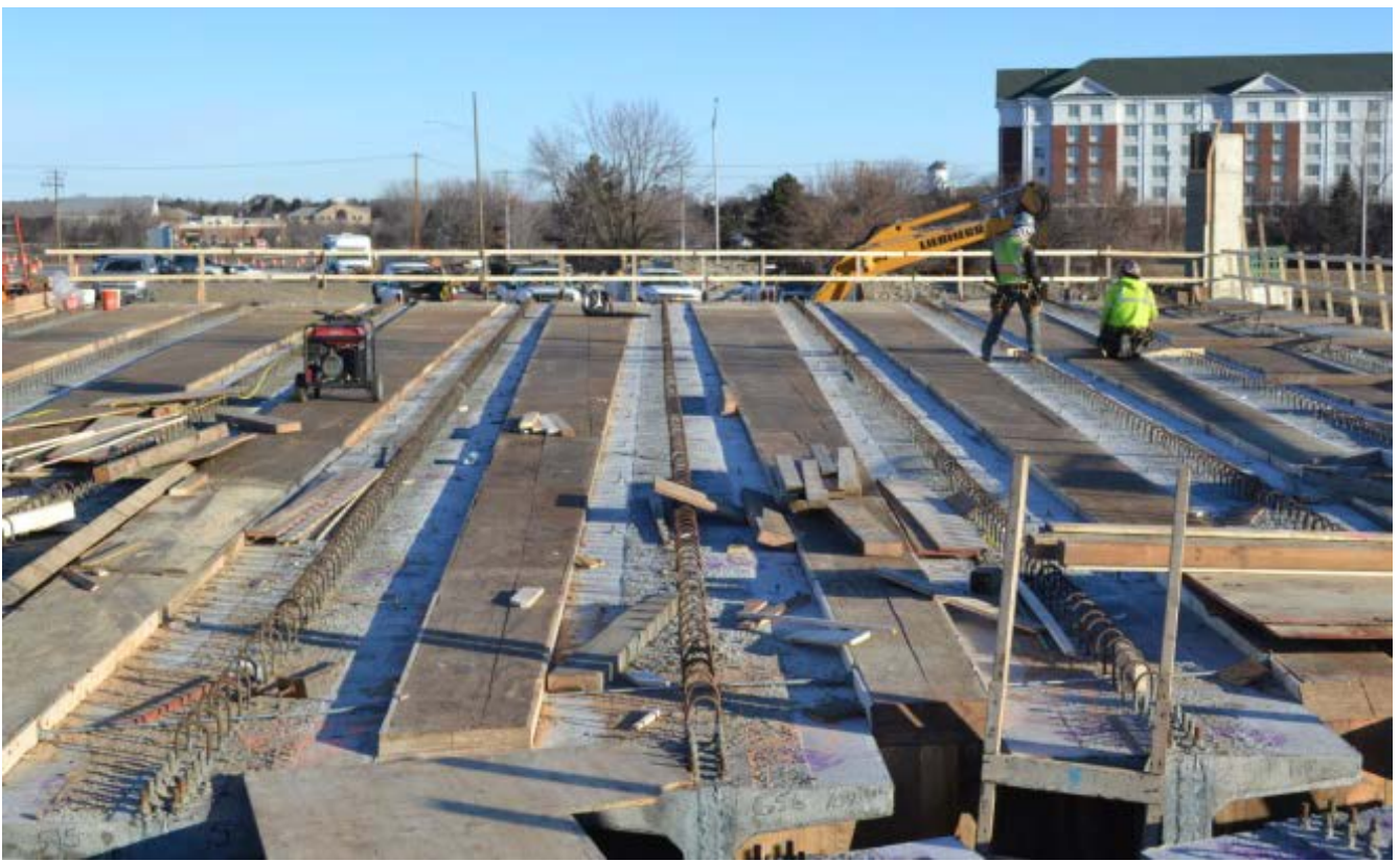
The false deck under construction. The fillets assured that the final position of the 8 inch deck was at the proper elevation.
