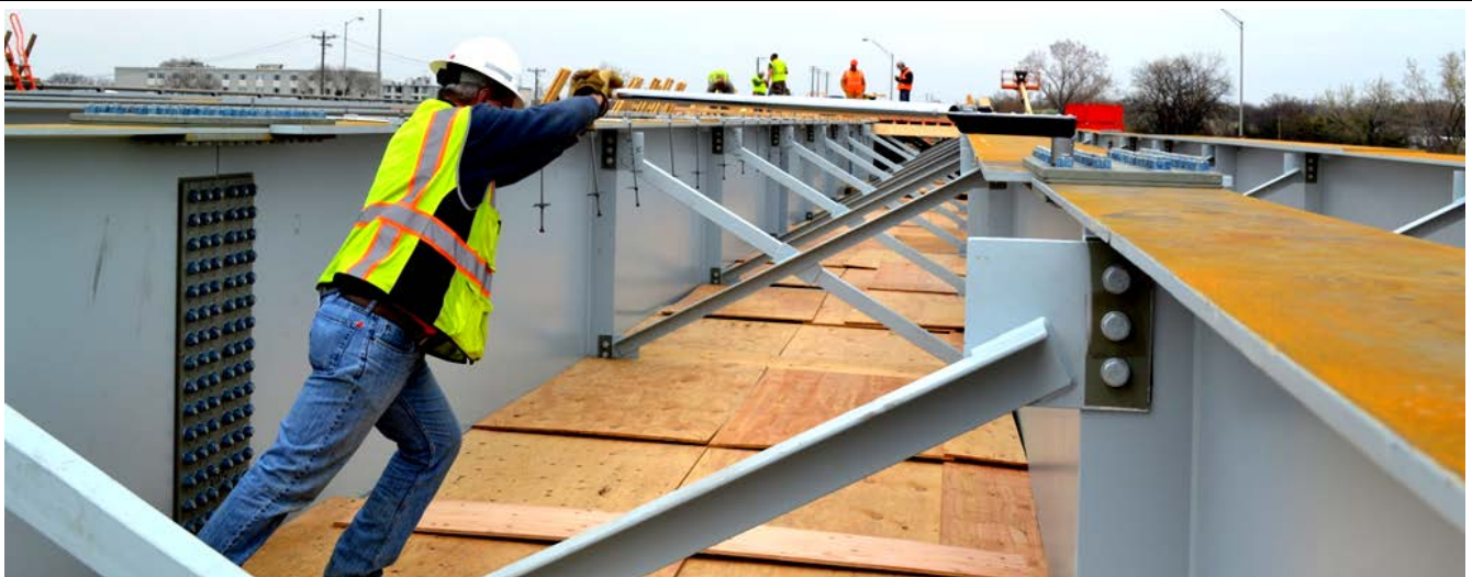
The CM Inspector testing a random flange bolt to verify that the proper torque was applied.
