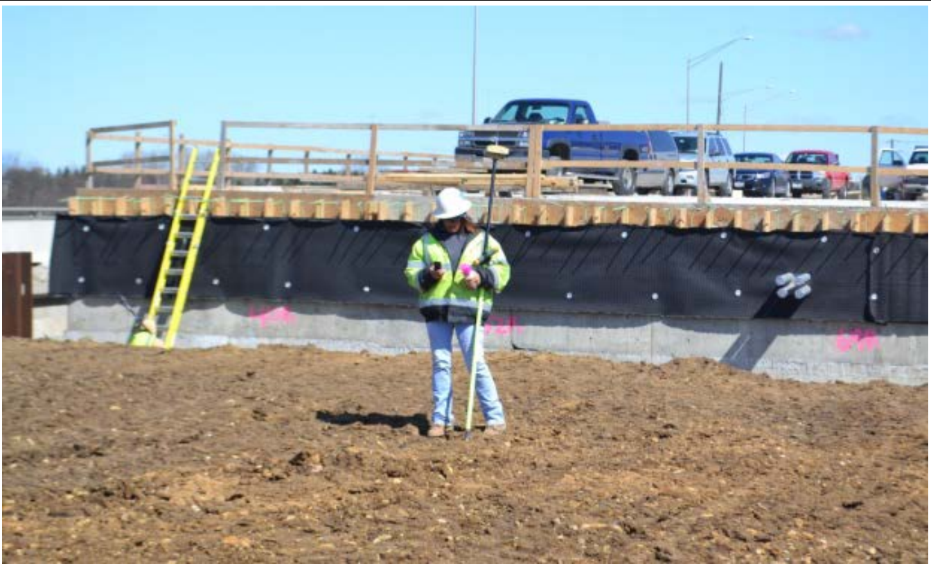
A surveyor with GPS takes measurements to verify the embankment elevation near the final surface.
