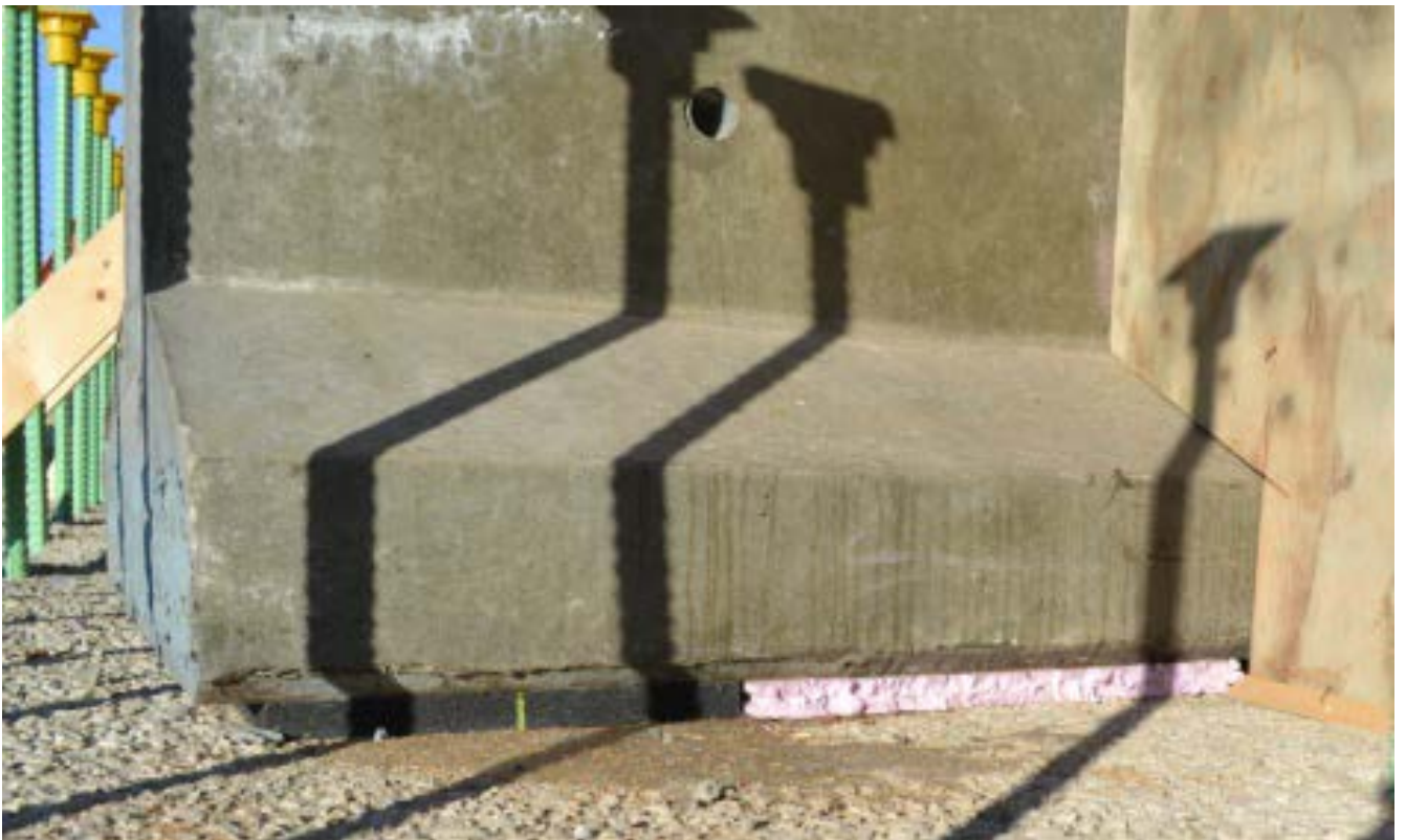
A fixed bearing for the concrete beam. This end will be buried into the concrete diaphragm.
