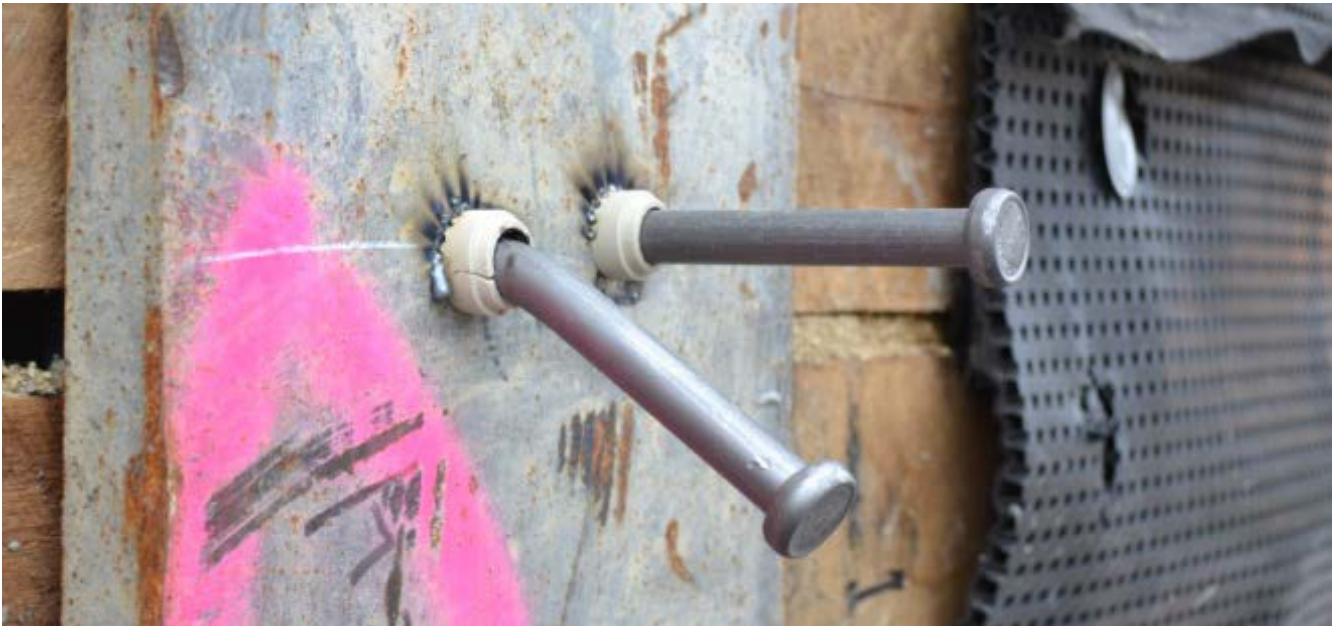
Stud shear connectors welded to soldier pile. The CM Team tested for proper connection by bending 45 degrees. “Just hit it real hard with a heavy hammer!”
