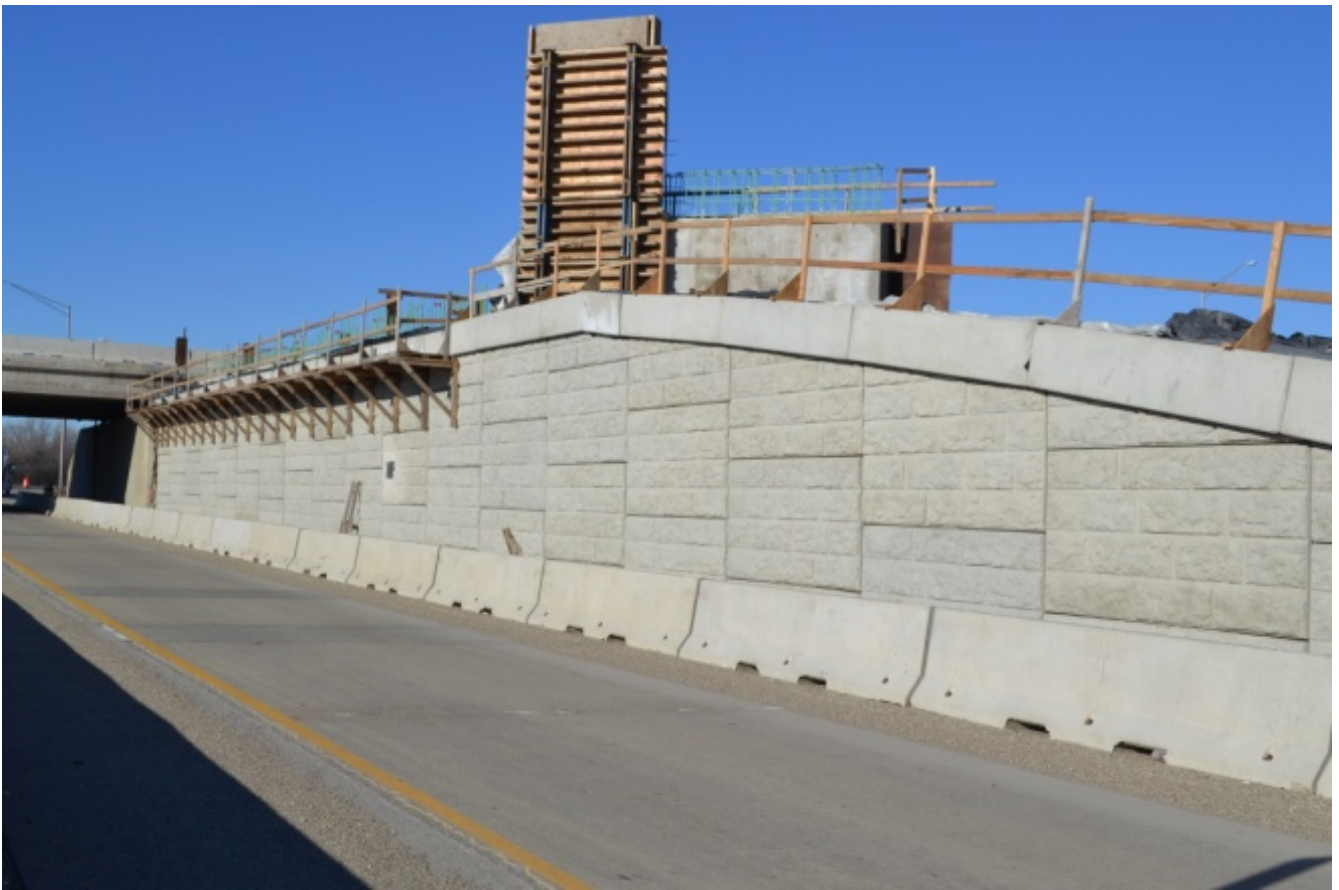
Front of MSE Wall with coping. Construction is nearly complete.
