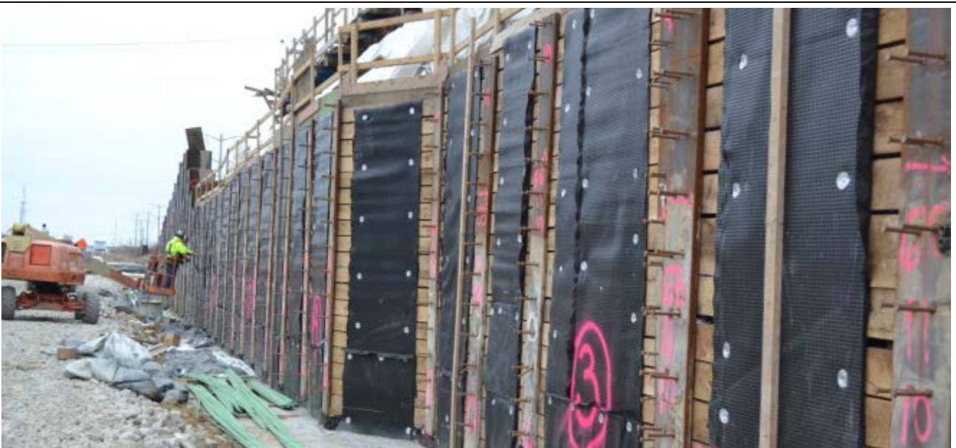
Soldier piles with stud shear connectors ready for re-bars, forms, and concrete.
