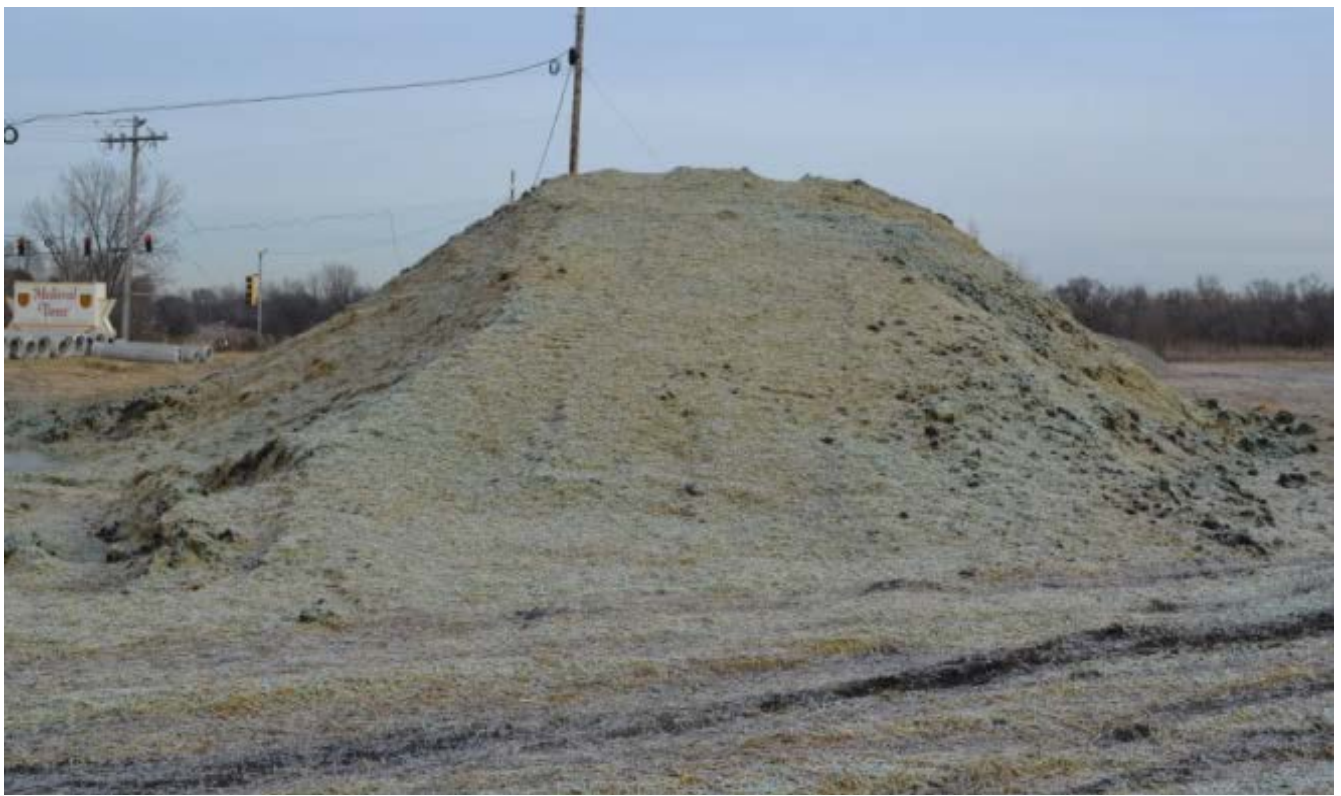
Topsoil stockpile seeded & blanketed. The seed is fast growing to provide erosion control as soon as possible.
