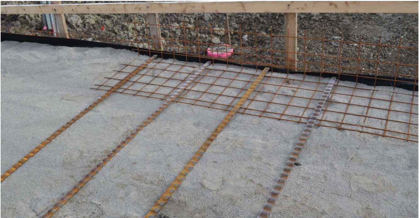
Temporary MSE Wall was completed with 18 inch baskets. Ties were buried in select backfill to provide support.
