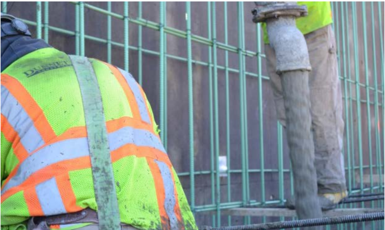
Concrete flowing from a concrete pump.
