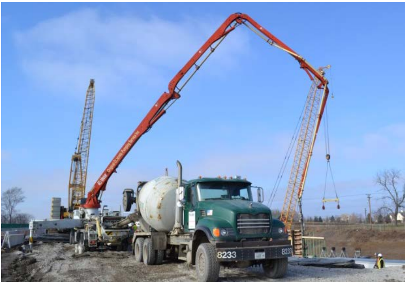
Concrete truck supplying 9 cubic yards and being pumped with a concrete pump.
