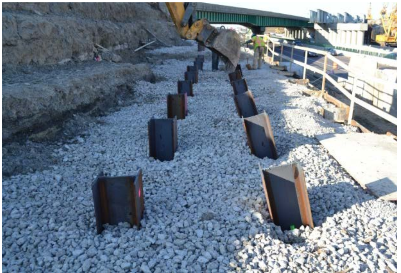
Abutment H-piles after select backfill was placed and cut off at the correct elevation .
