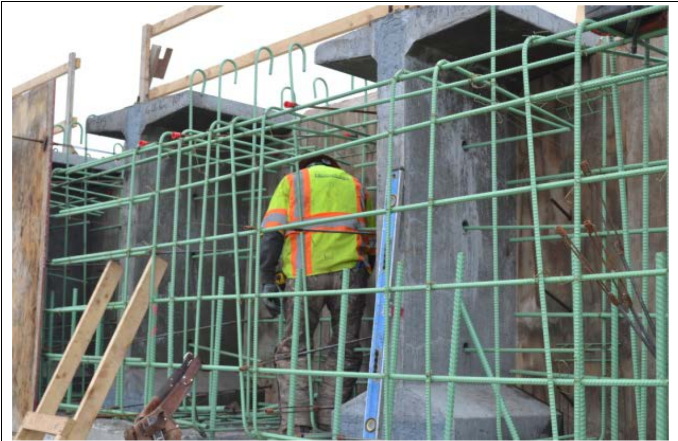
Epoxy coated re-bars were extended into the diaphragm and are ready for the forms and concrete.
