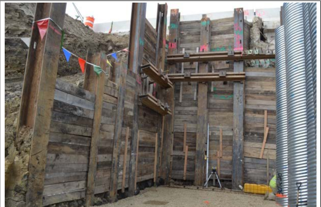
Soldier piles and lagging to transition from the existing sloped embankment.
