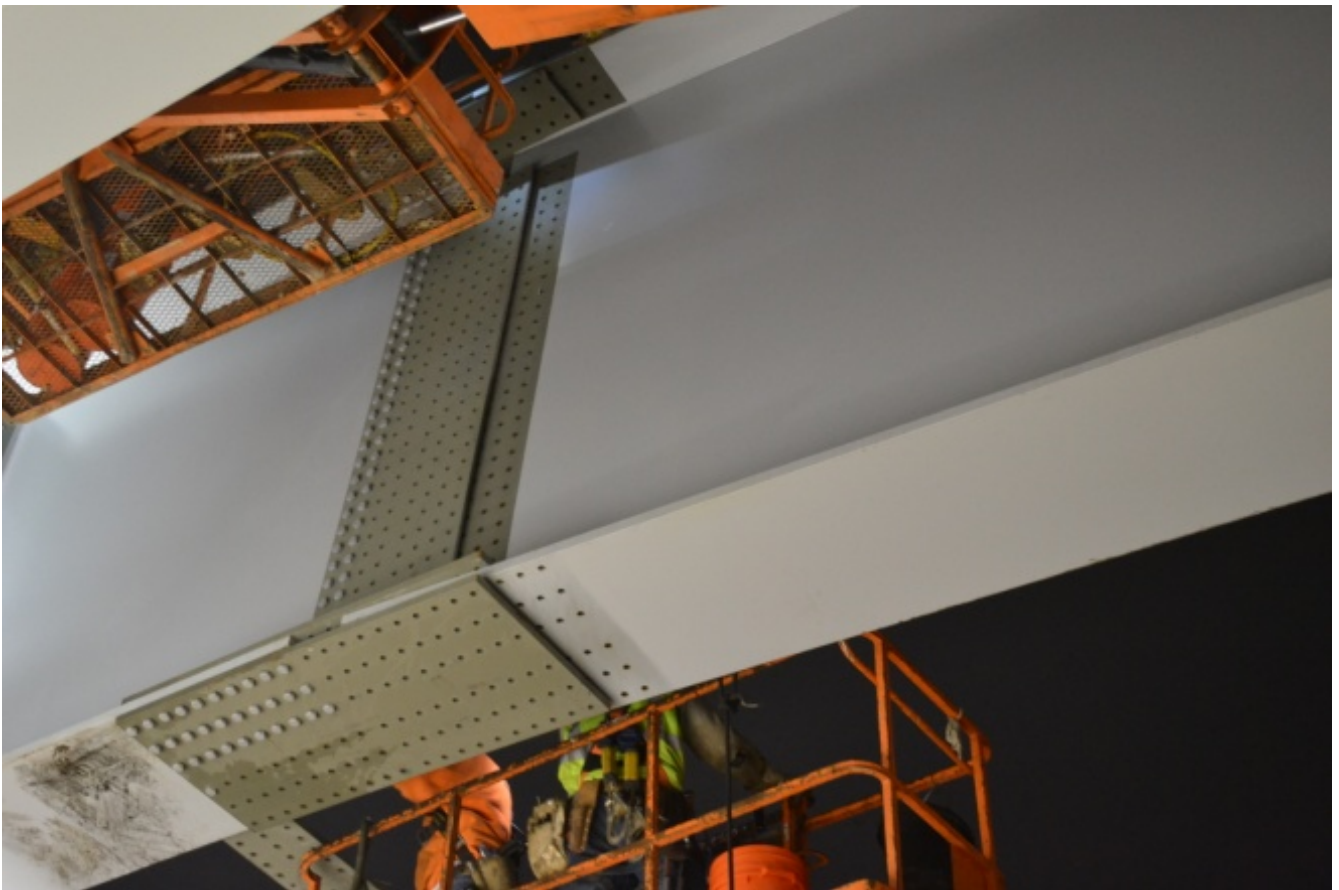
Beam being connected at a splice. The CM Team verified that a bolt was placed in each hole and was correctly tightened.
