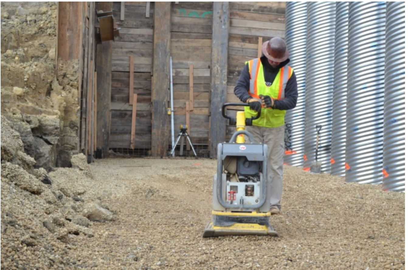
Select backfill being placed, graded, and properly compacted.
