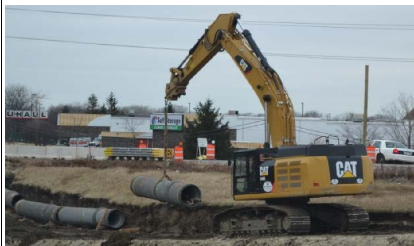
Water line being relocated. Engineers will pressure test to verify no leaks and test for water purity after installation. The CM Team will mark the new route on the as built plans.
