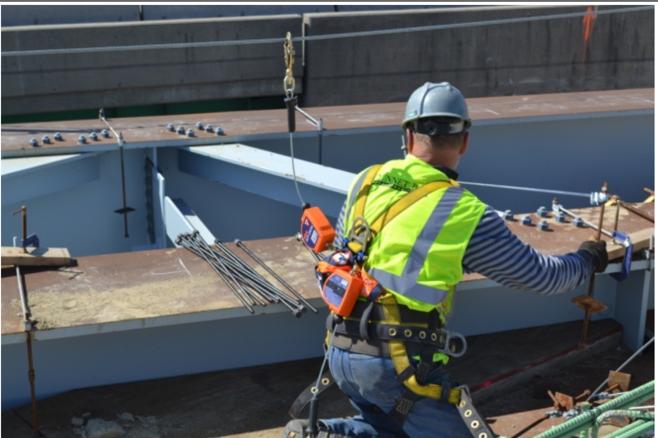
When a beam was more than 6 feet deep, OSHA requires the worker or inspector to be “tied off” to prevent falling. This is the correct equipment and method.
