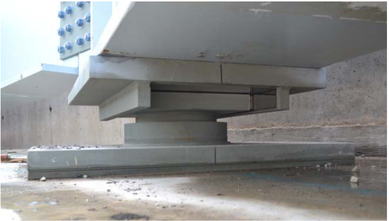
Multi-rotational disc bearing on an abutment for the movable end. It was designed to allow the beam to slide and rotate.
