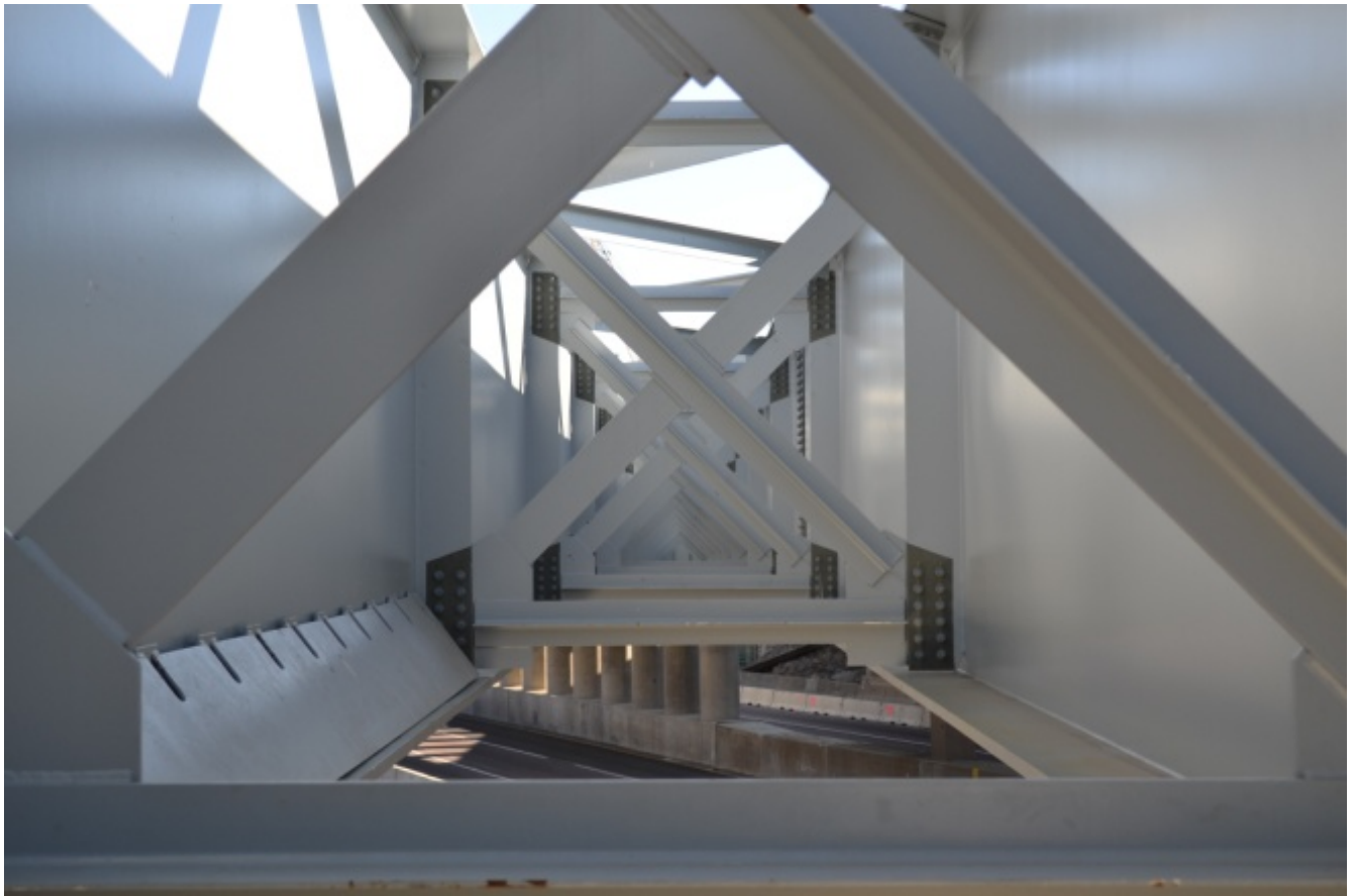
Cross members bolted to the beams.
