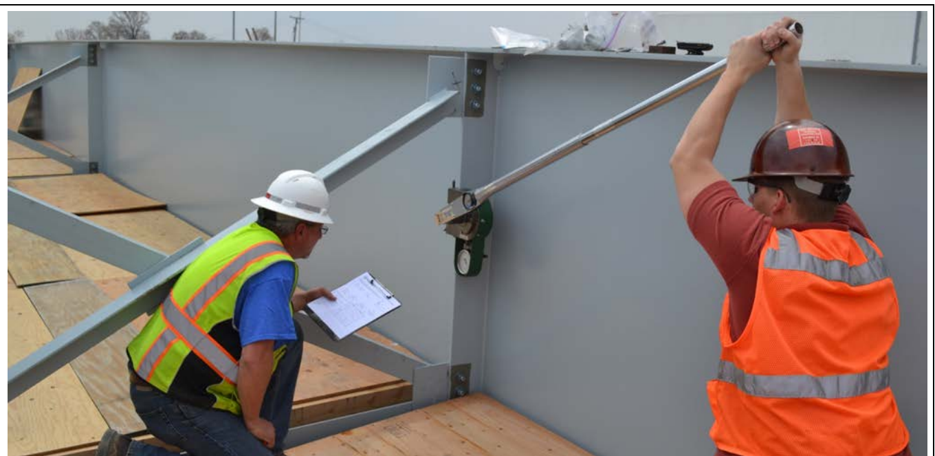
The CM Inspector and contractor testing bolts to verify a torque of 50,000 ft-pounds force before breaking or stripping.
