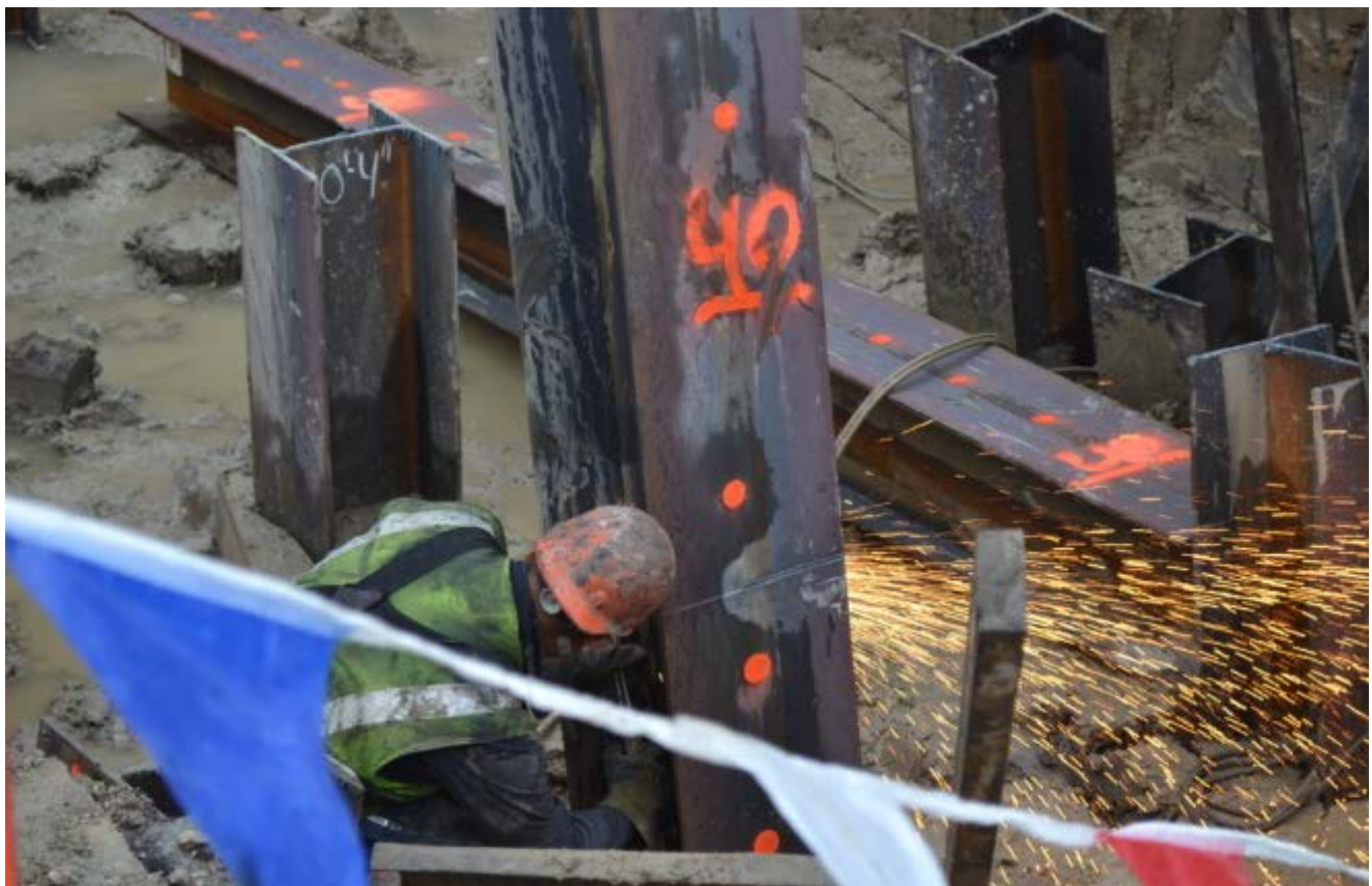
Engineers marked the correct final top of pile elevation and the excess was cut off.
