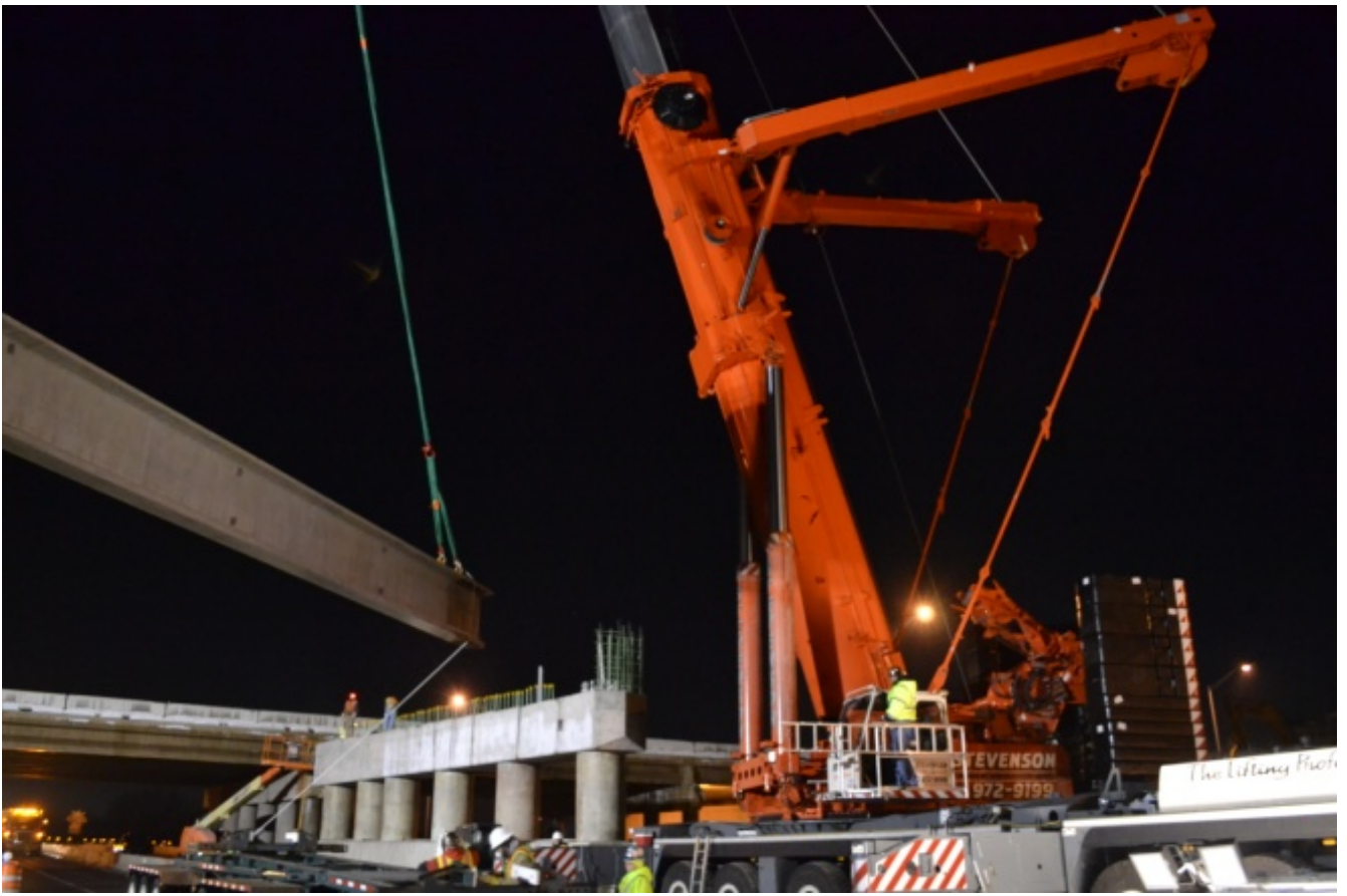
The contractor used a 600 ton crane with a 164 foot boom. All of this equipment was designed by engineers.
