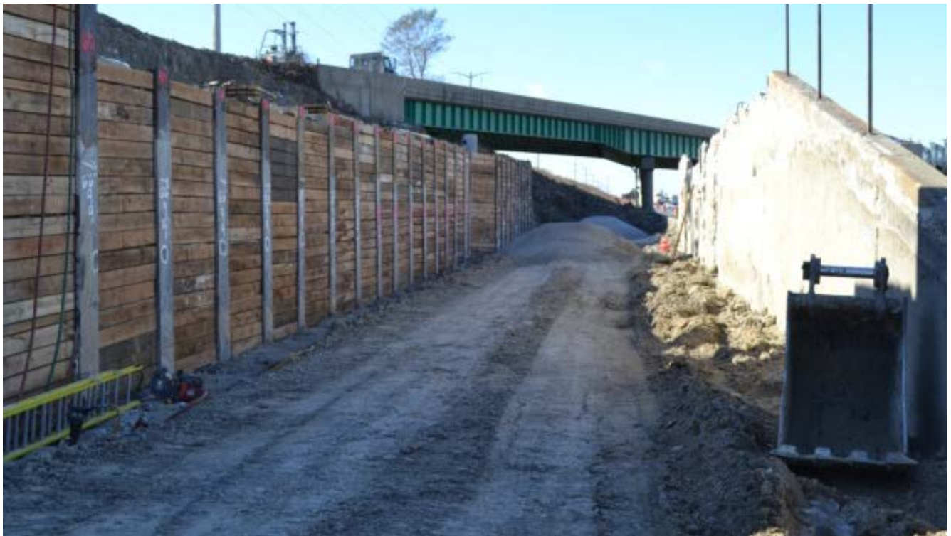
Temporary Retaining Wall constructed with soldier piles and lagging.
