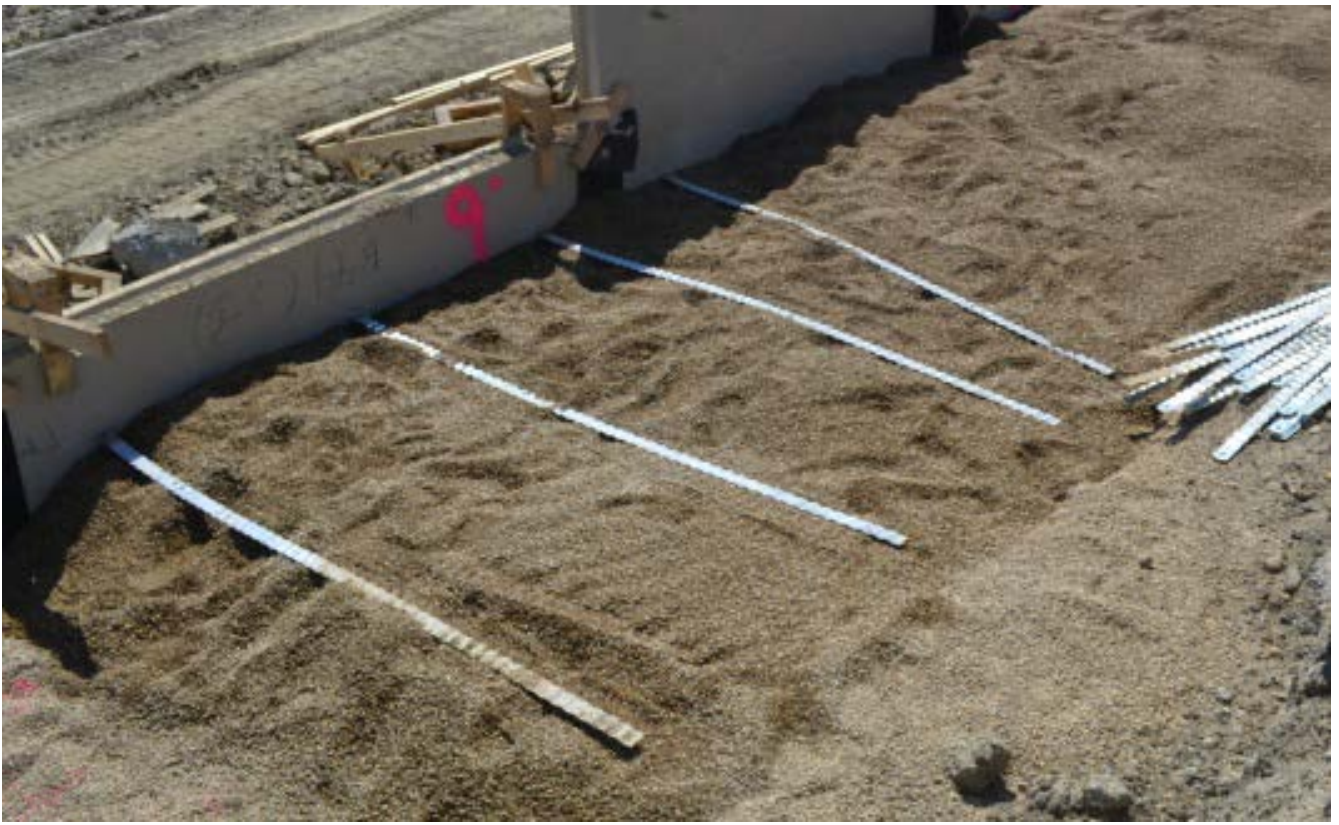
Tieback straps properly spaced to support the wall and ready to be covered with select backfill.
