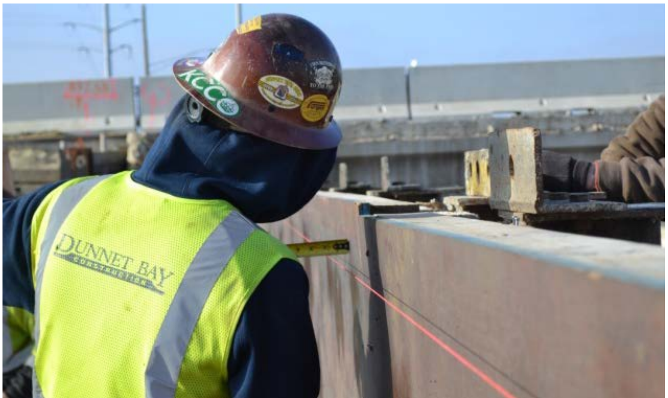
Contractor making a final measurement to verify proper form position.
