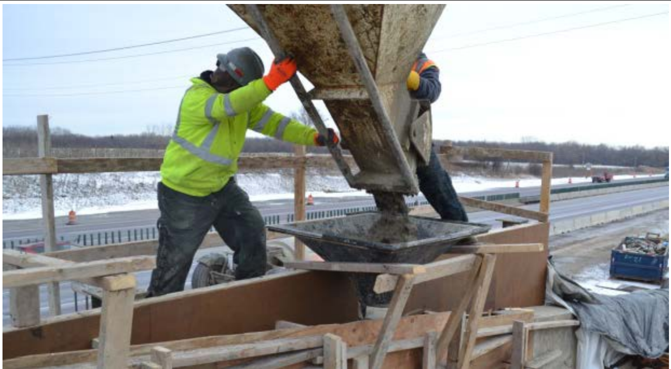
Pouring concrete with a bucket. When concrete must fall more than 6 feet, it must be installed with a chute. The CM Team verifies proper concrete placement.
