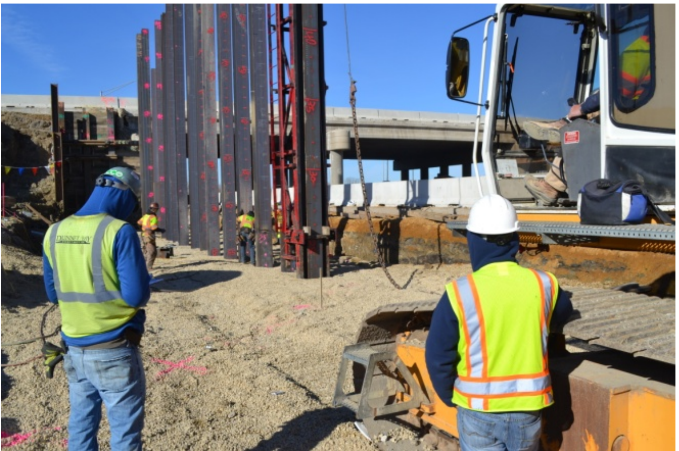
QC and QA Inspectors counting blows per foot during pile driving. They solved the following calculation to determine that the pile reached the proper depth.
