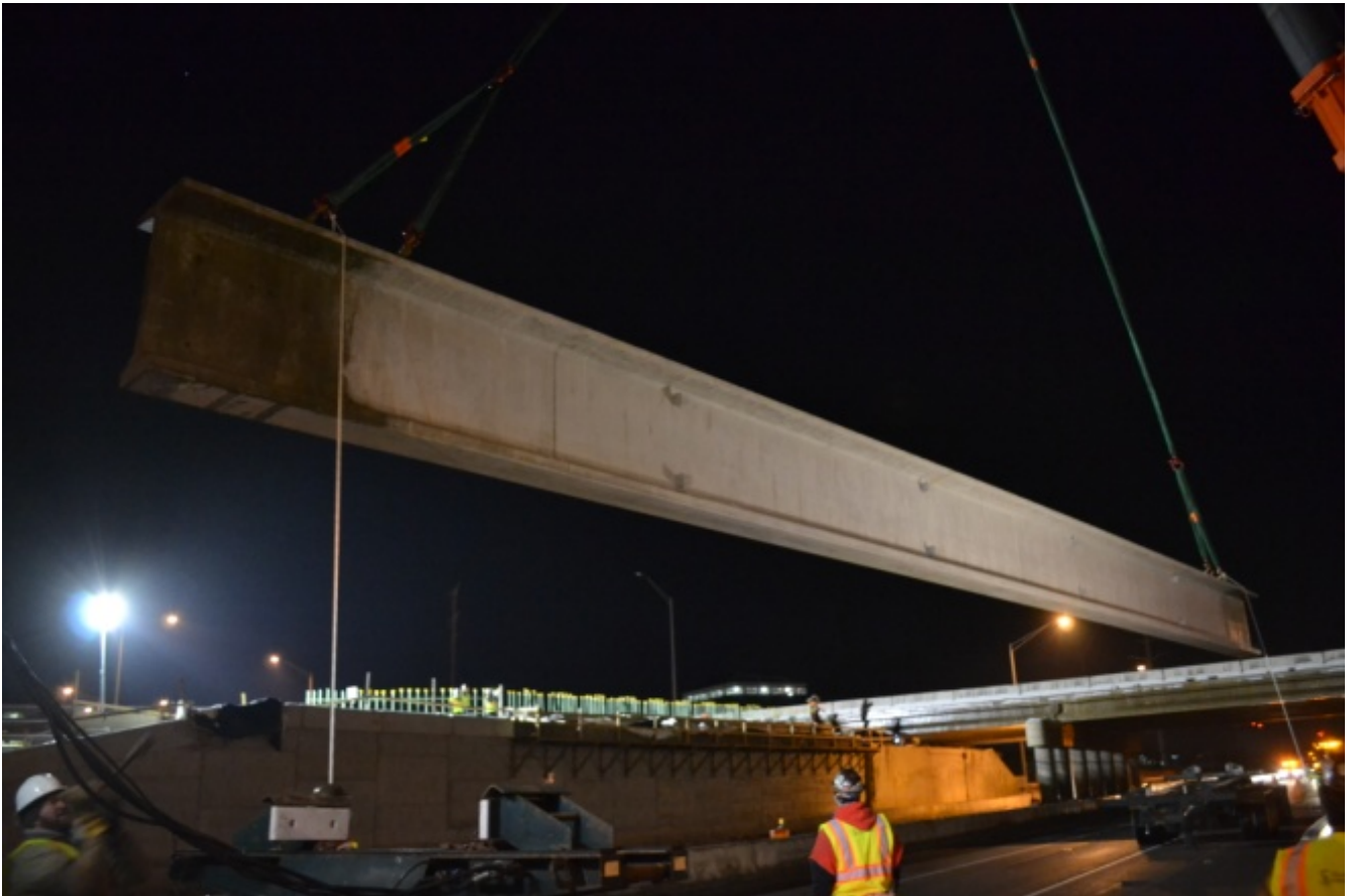
The beam being lifted to straddle from abutment to pier.
