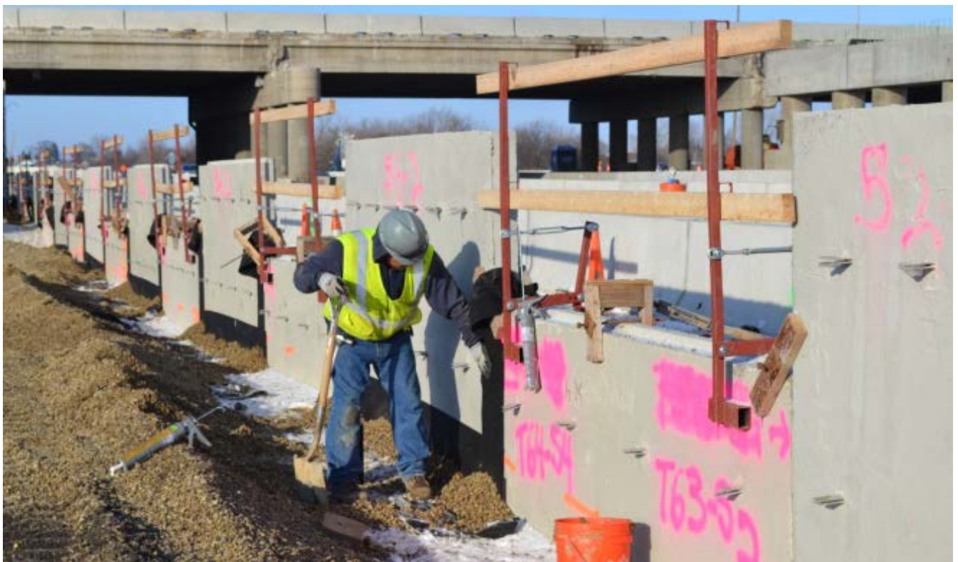
The rear of the MSE Wall during installation.
