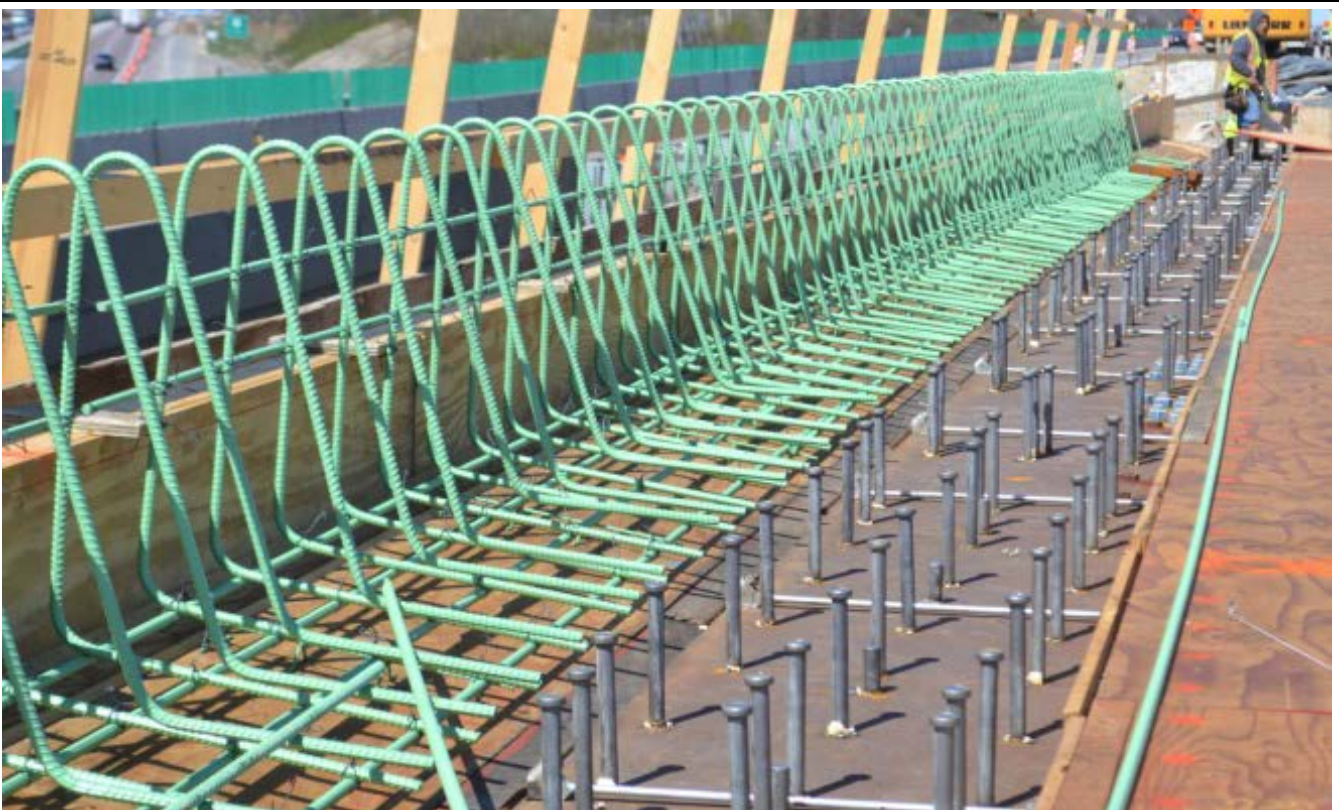
The barricade wall was constructed integral with the deck.
