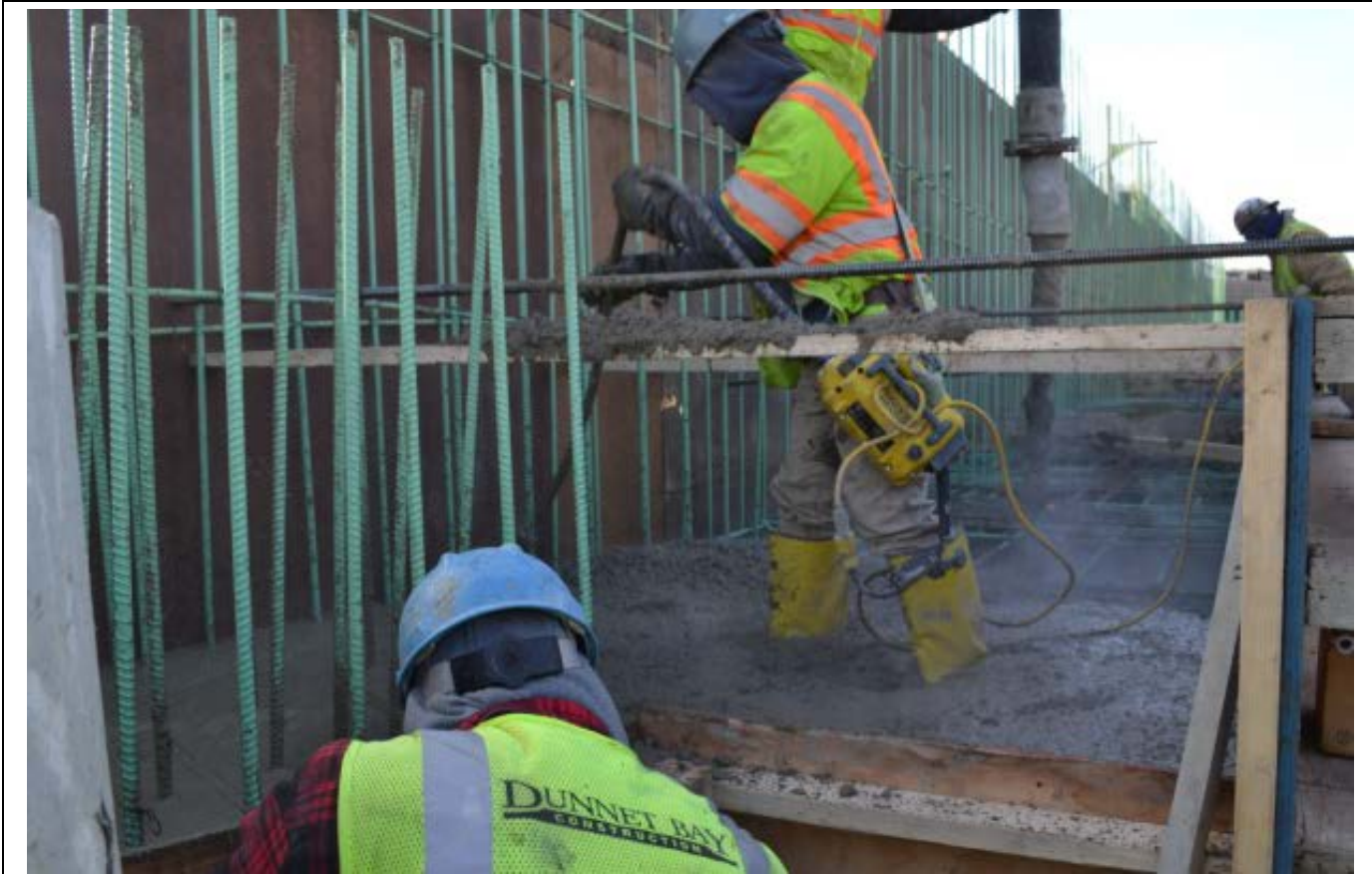
Concrete being placed into the abutment.
