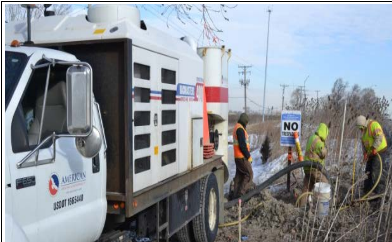
Engineers searching for a high pressure petroleum line with a vacuum excavator. The CM Team will mark the depth and location on the as built plans.
