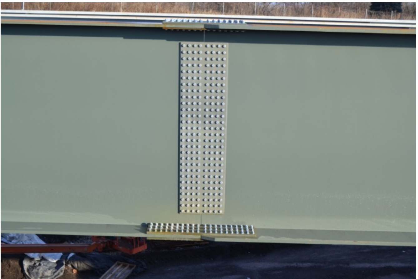
Splice plate and bolts on top flange, bottom flange, and web.
