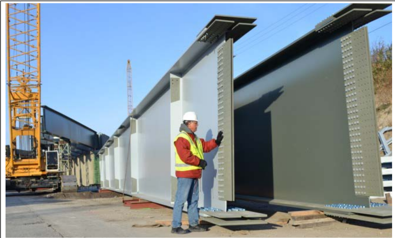
Steel beam, 10 feet (H) by 110 feet (L).
