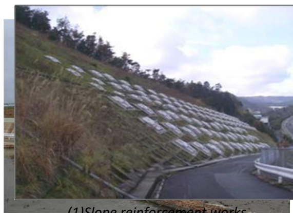
(1) Slope reinforcement works
