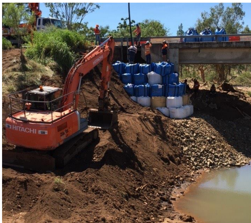
Figure 4.3.2.4 Granite Creek Bridge repair
