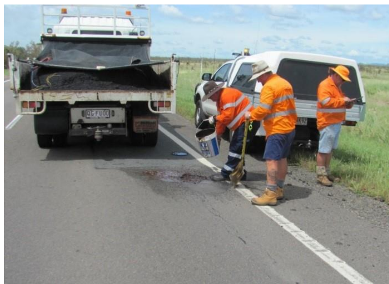
Figure 4.3.2.5 TMR crew pothole patching and updating RADAR near Rockhampton
