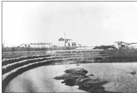
**Figura 2. First work in wire gabions**
