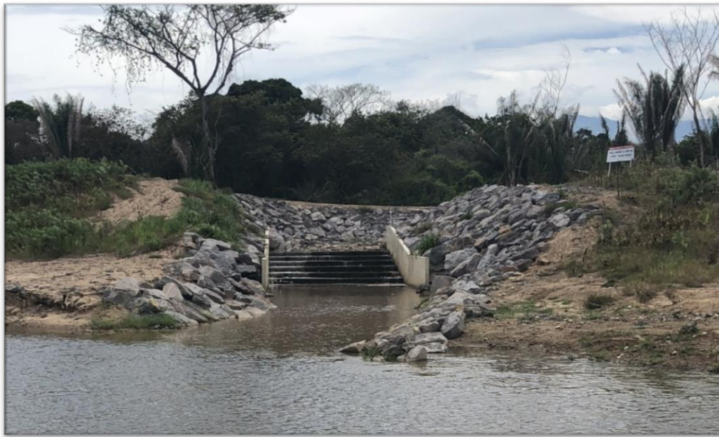
Figure 2. Stepped structure with skimming flow for the Caño Piedras-La Loma, Cesar
