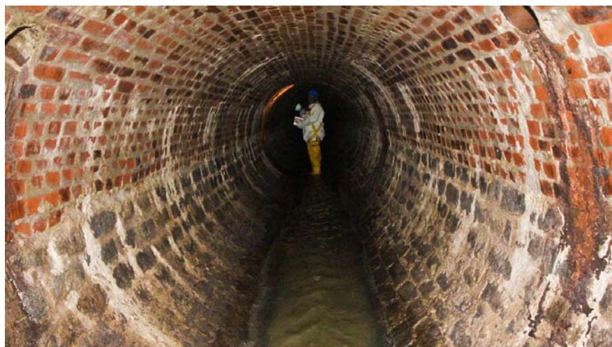
FIGURE 1.1 Brick sewers built in Philadelphia, some of which are nearly 200 years old, are still in use today. SOURCE: Photograph by Kimberly Paynter.
