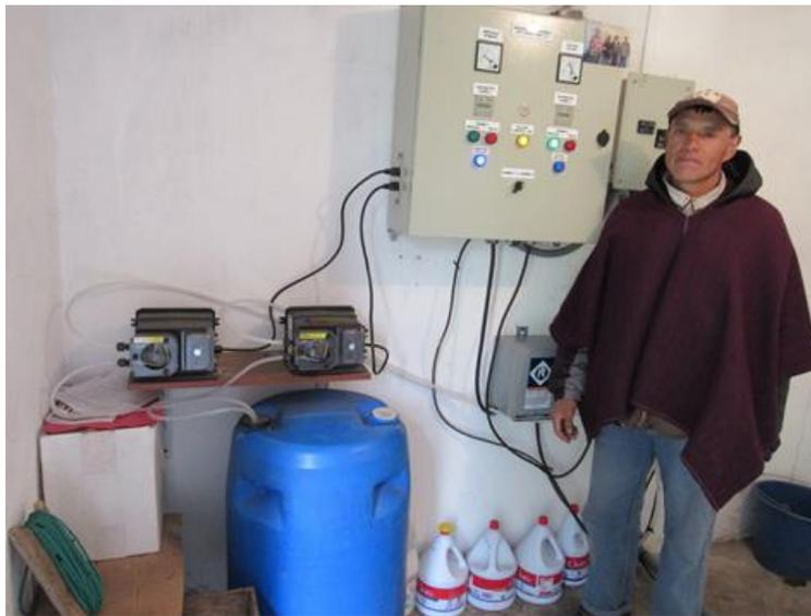
*Figure 6 Water system operator for Achullay and electrical panel controlling the water supply and chlorine dosing pumps. Note the two peristaltic dosing pumps, one for each water supply pump, and the blue chlorine solution feed tank.*
