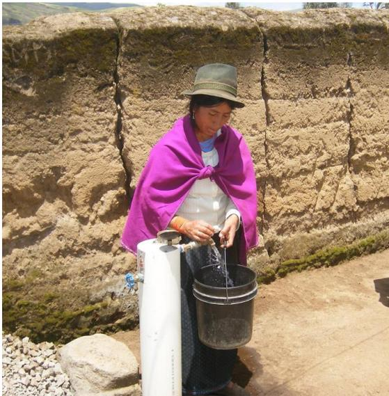
*Figure 1 Typical concrete pedestal mounted metered spigot for a Kichwa home*
